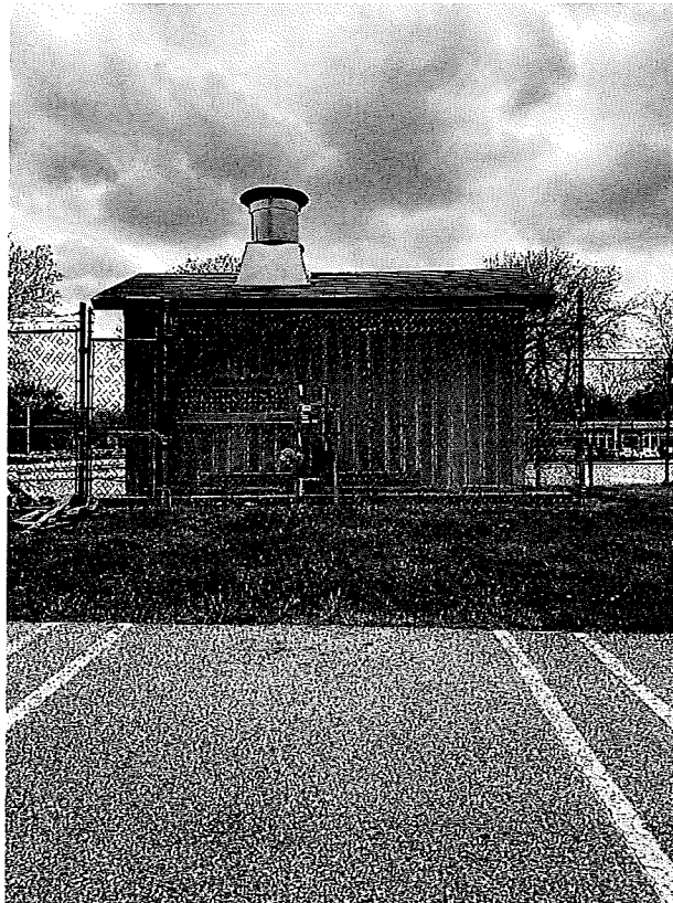
Back of Heater Shed
