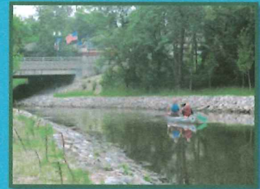
Mayor Haidous of Wayne canoees down the Rouge River after completion of the Wayne Road Dam Removal and Restoration Project funded through the National Oceanic and Atmospheric Administration
