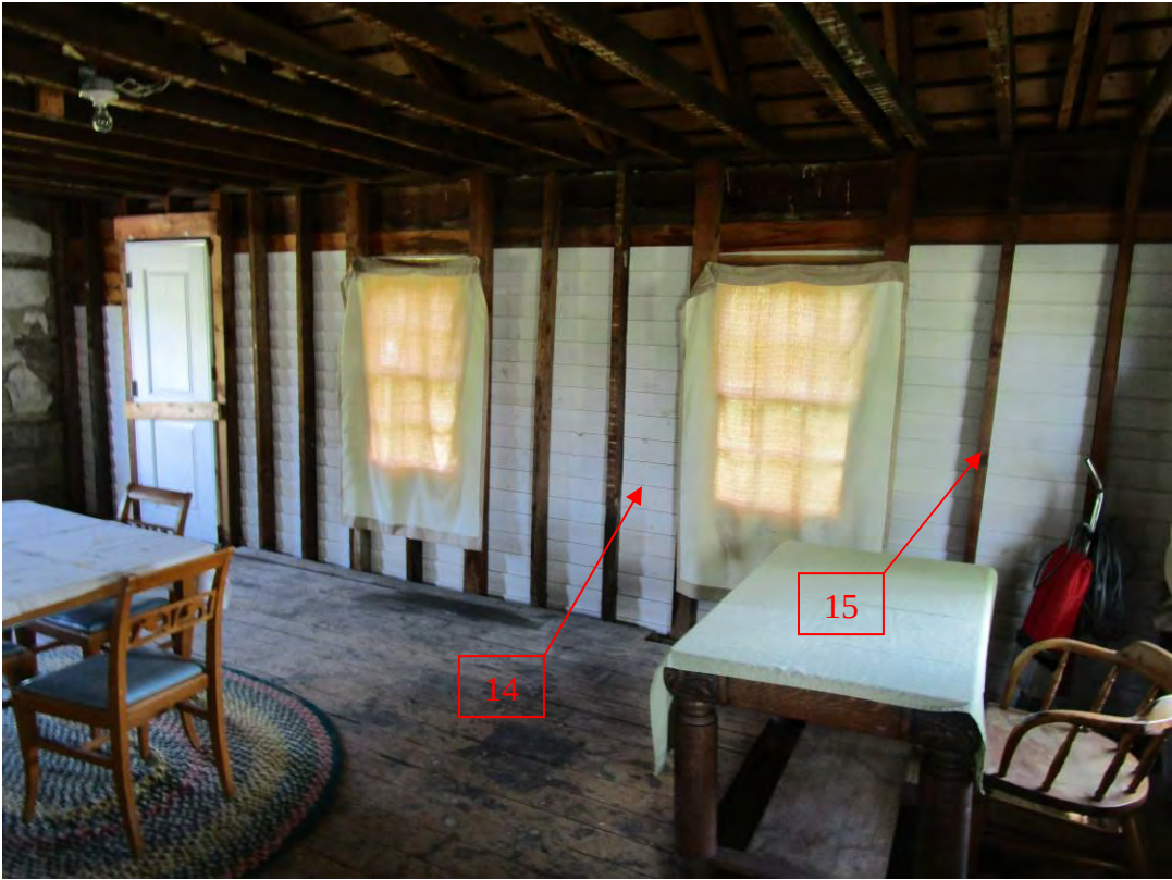
Interior Looking East
