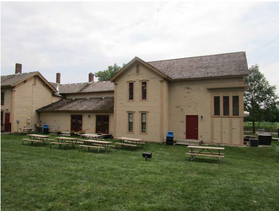
Partial North Elevation
