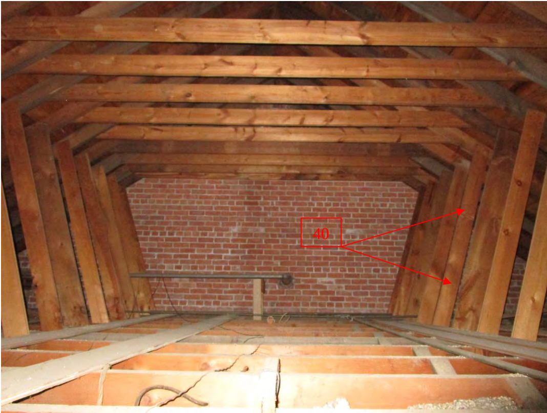
Attic Looking North
