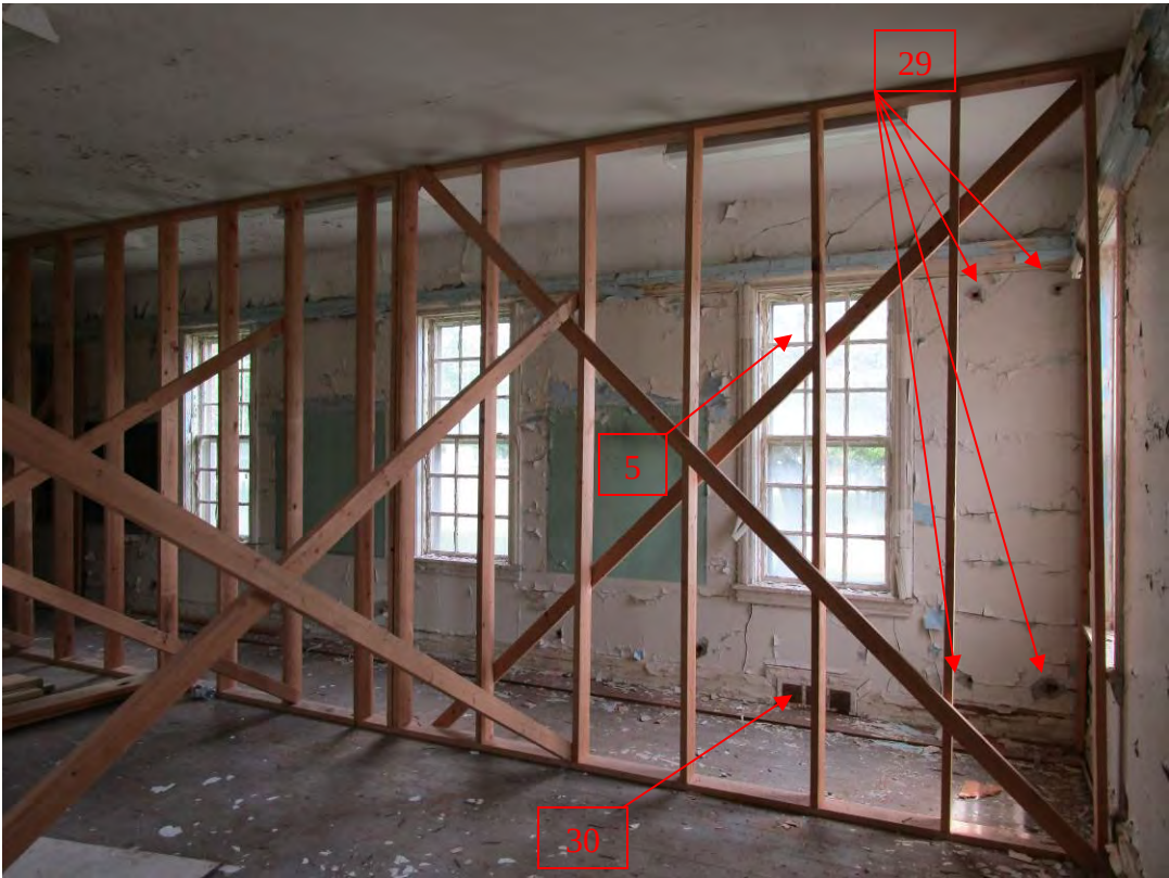
Interior Looking East
