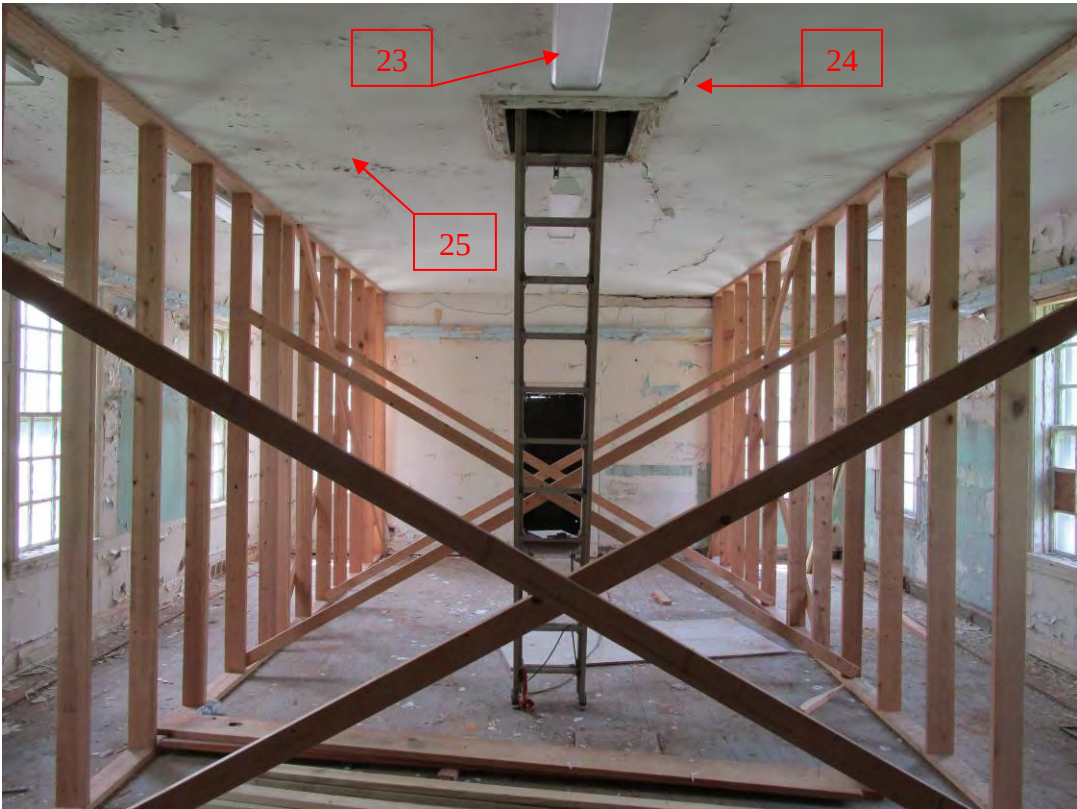
Interior Looking South
