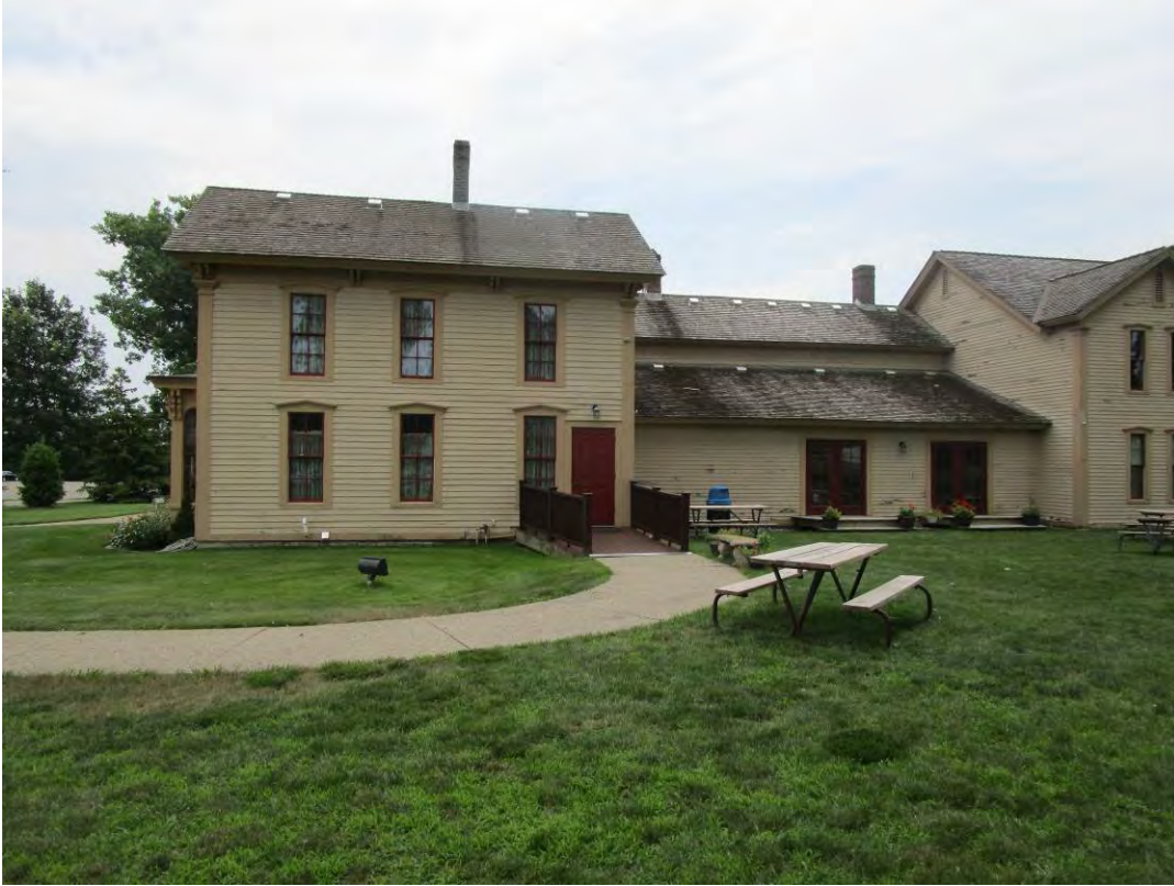
Partial North Elevation
