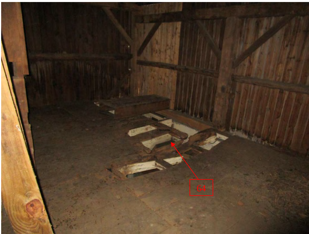
East Elevation Detail Northwest Corner (Bay 1)
