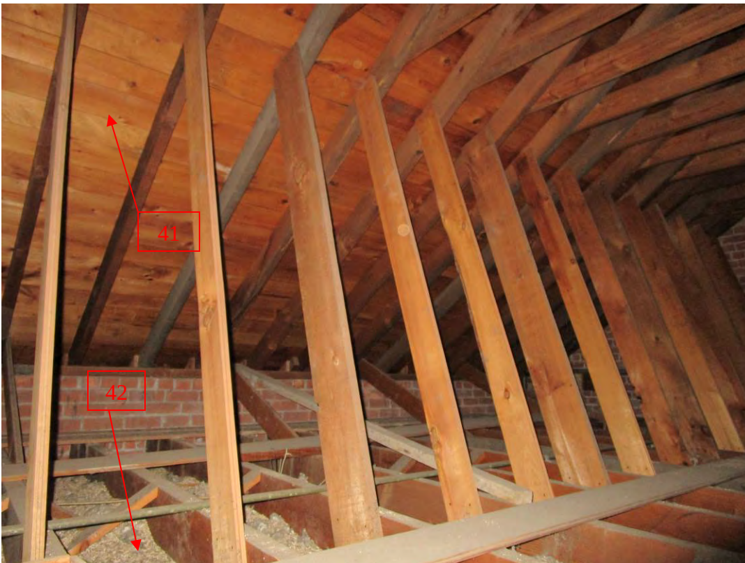
Attic Looking Northwest
