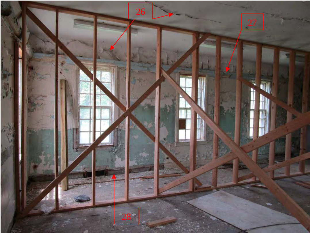
Interior Looking West
