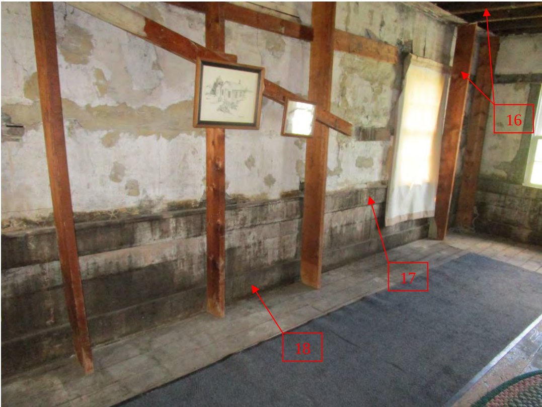
Interior Looking West
