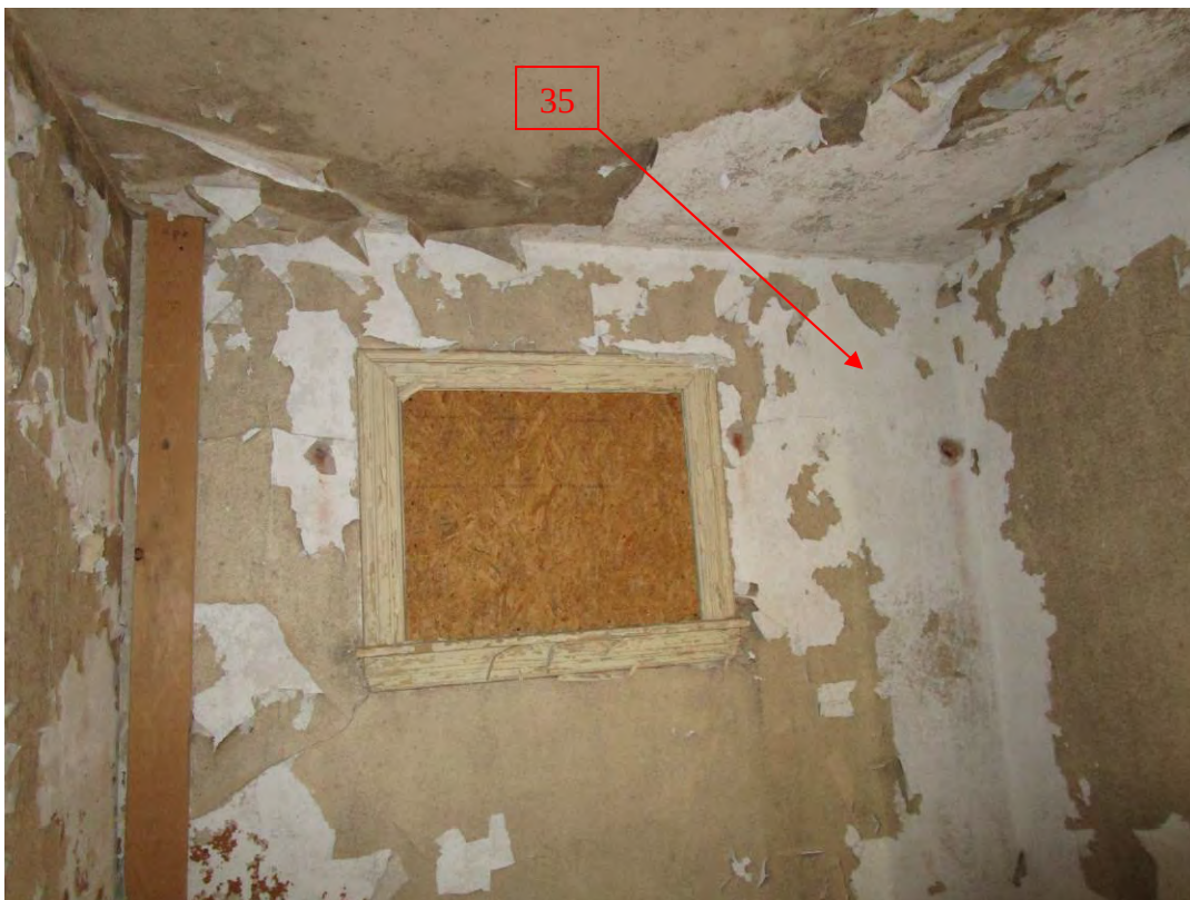
Vestibule Looking East
