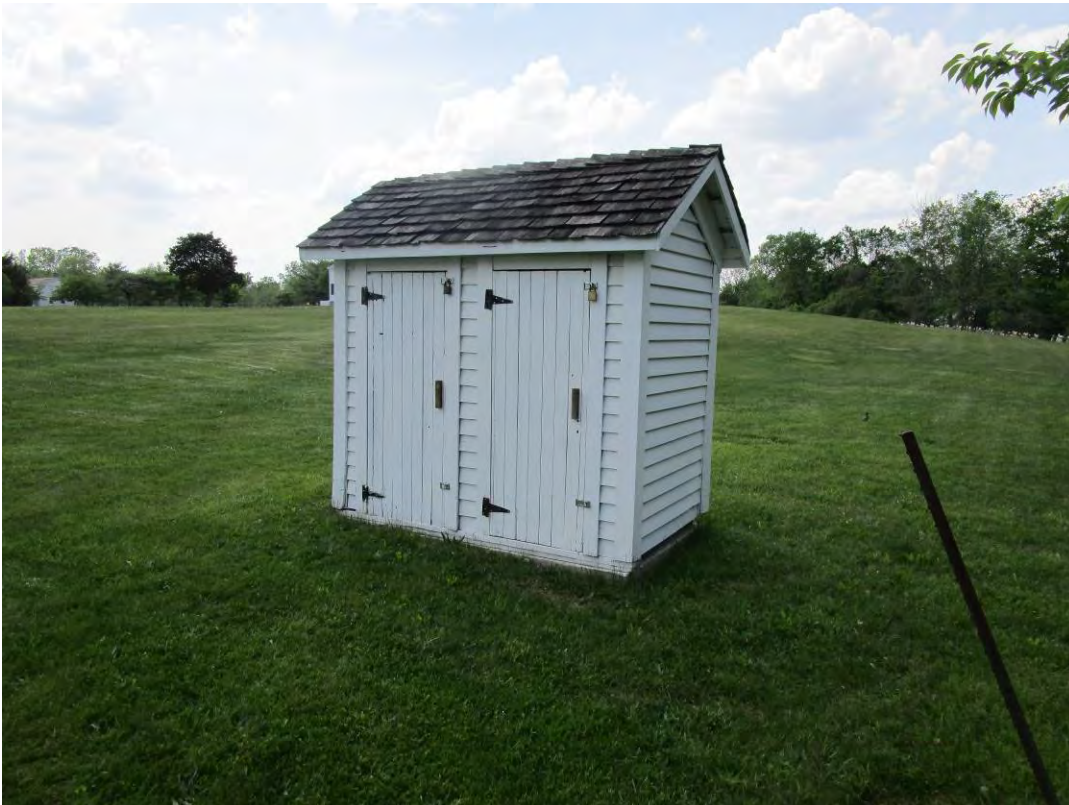
Outhouse East Elevation
