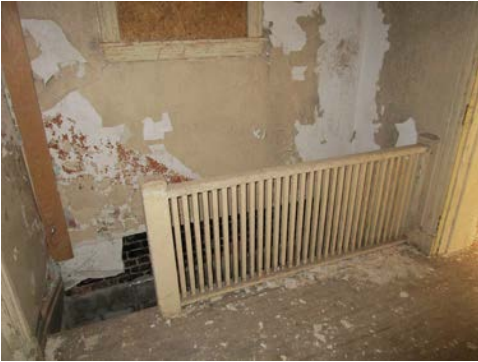
Stairwell Opening Into School Basement
