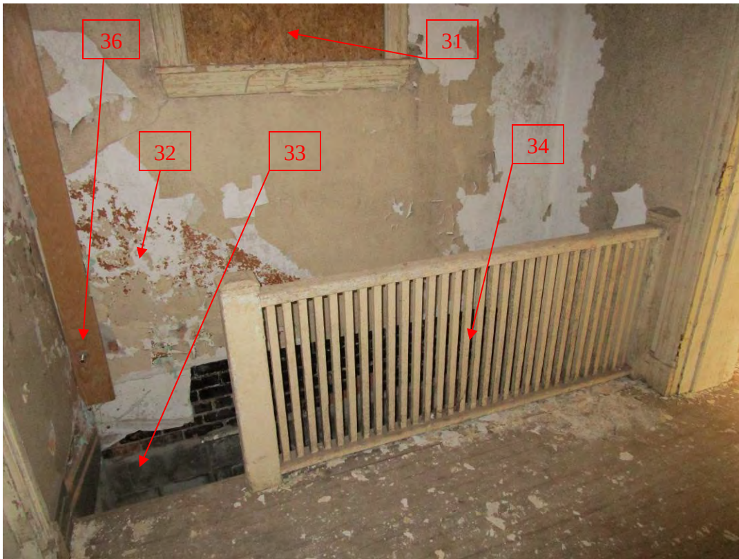
Vestibule Looking West at Access to Basement
