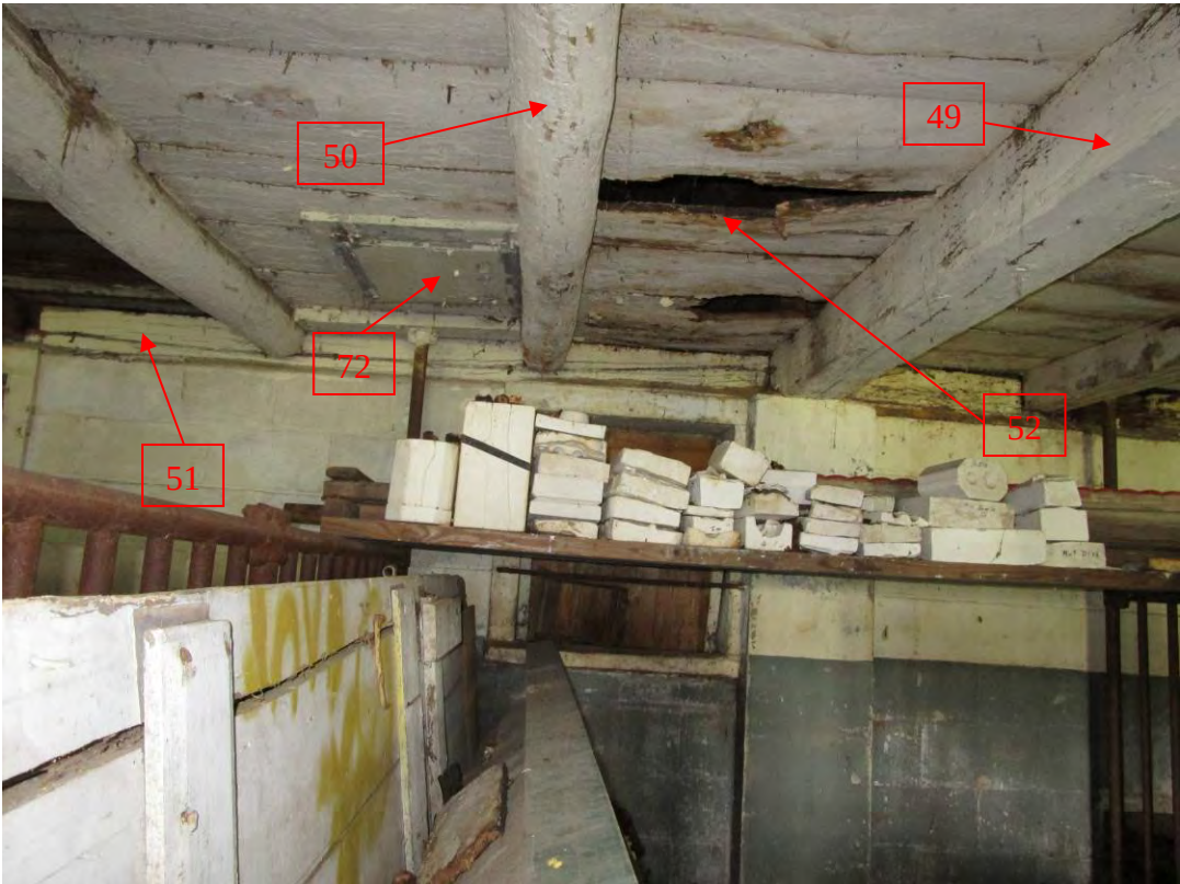
East Elevation Detail Looking West
