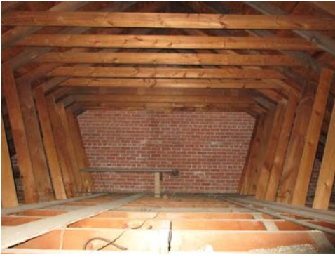
Attic Bracing for the 2016 Building Move
