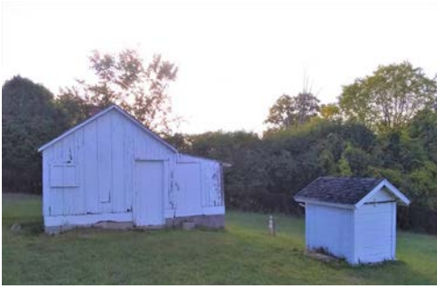
Outbuildings at the Shaw House
