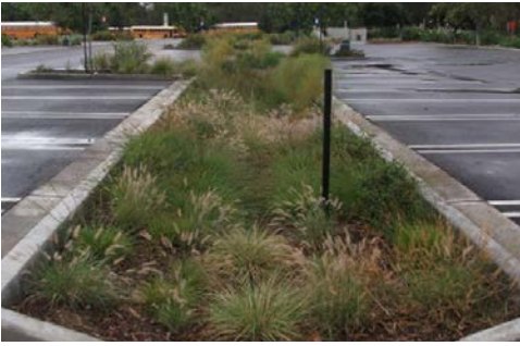
Example of parking lot bioswale - MSU Extension
