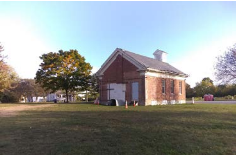
Rear Elevation of the Nankin Mills School
