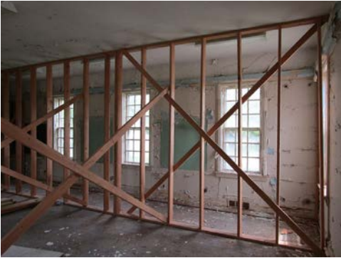
Interior bracing Looking East
