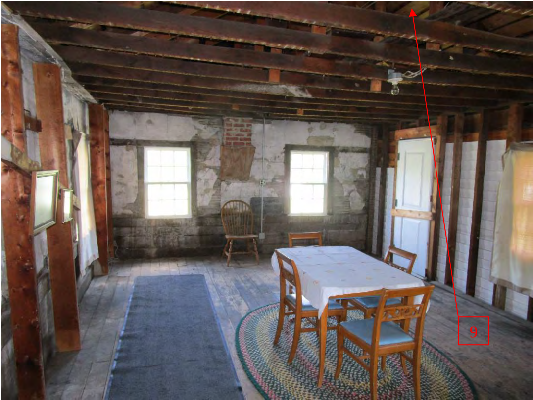
Interior Looking North
