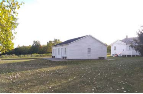
Village Print Shop - Constructed 2003 Building is proposed to be repurposed and enlarged for the Collections building
