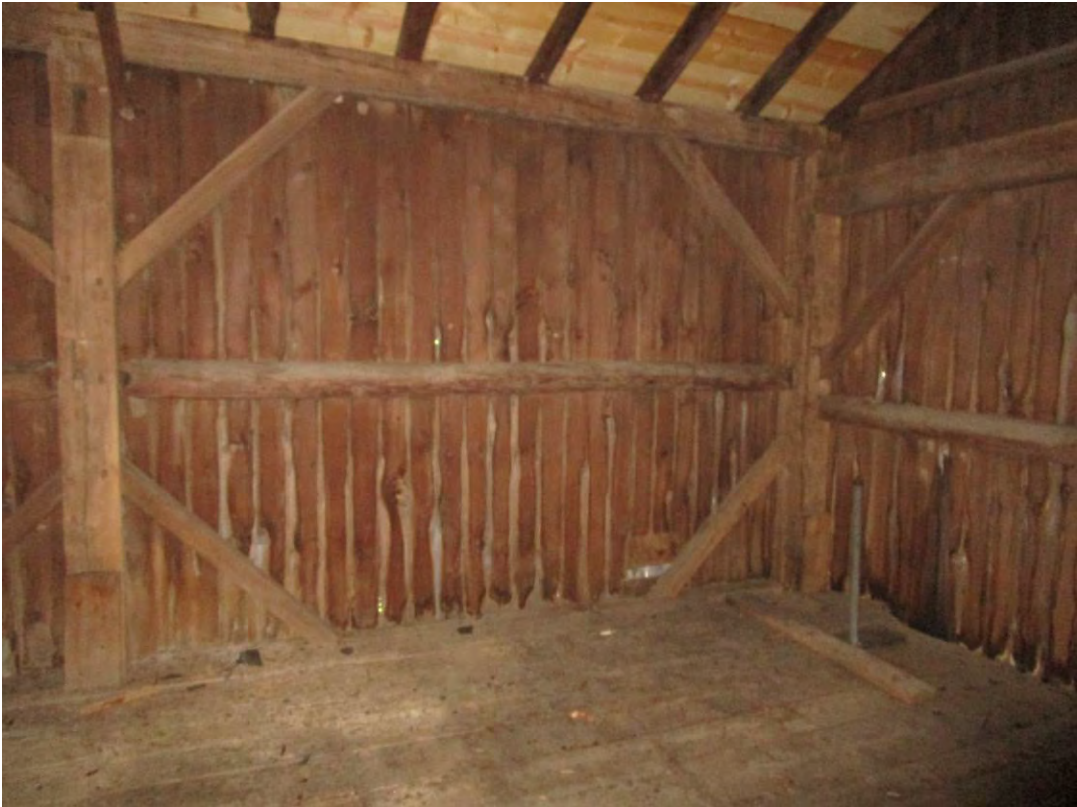
East Elevation Detail Southeast Corner (Bay 5)
