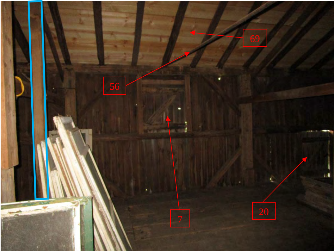
East Elevation Detail Looking East (Center Bay)
