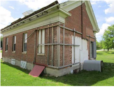
Exterior Bracing at Northeast Corner
