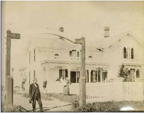
Historic Entry Gateway - Alexander Blue House Courtesy of Greenmead Historical Park
