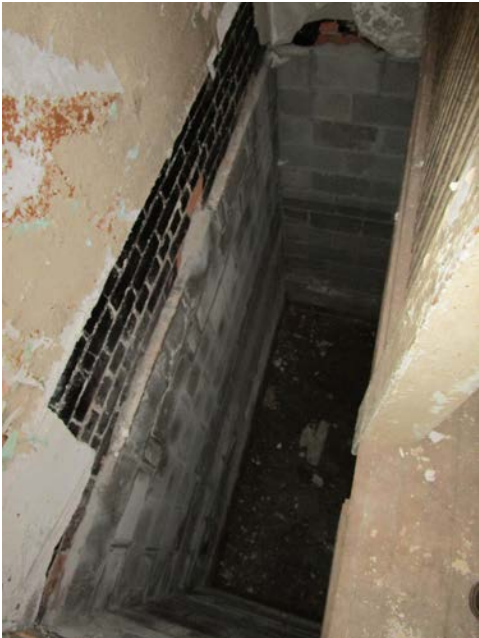
Opening for Basement Stairs
