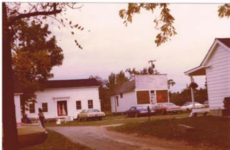
Shaw and Geer structures at Quaker Acres Courtesy of Greenmead Historical Park
