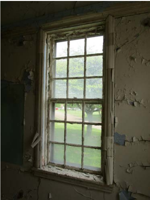
Interior Window Detail
