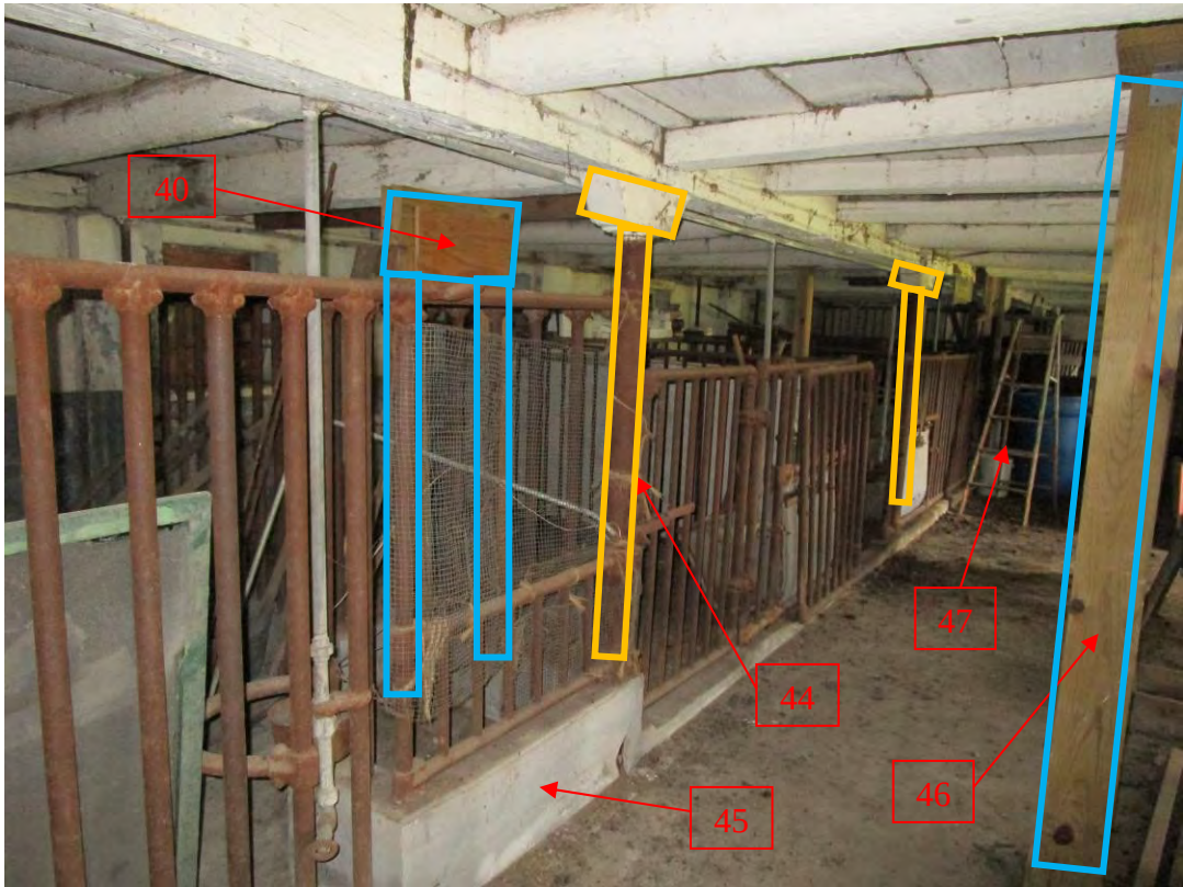
East Elevation Detail Looking Northwest
