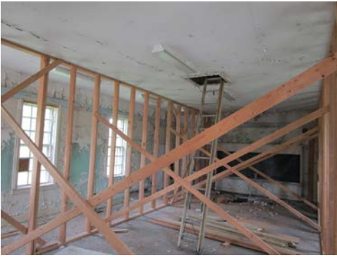
Interior Bracing Looking Northwest with Attic Entry
