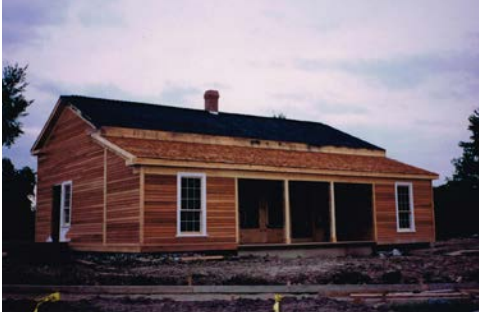
Meeting House - Under Rehabilitation Courtesy of Greenmead Historical Park
