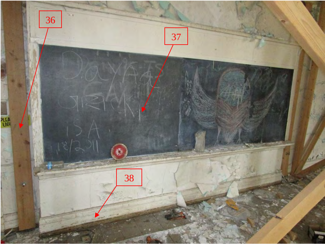
Interior Looking West at Chalkboard
