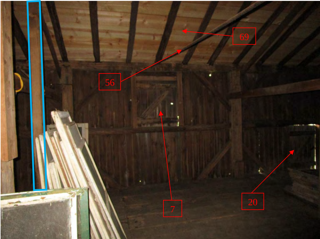
East Elevation Detail Looking East (Center Bay)
