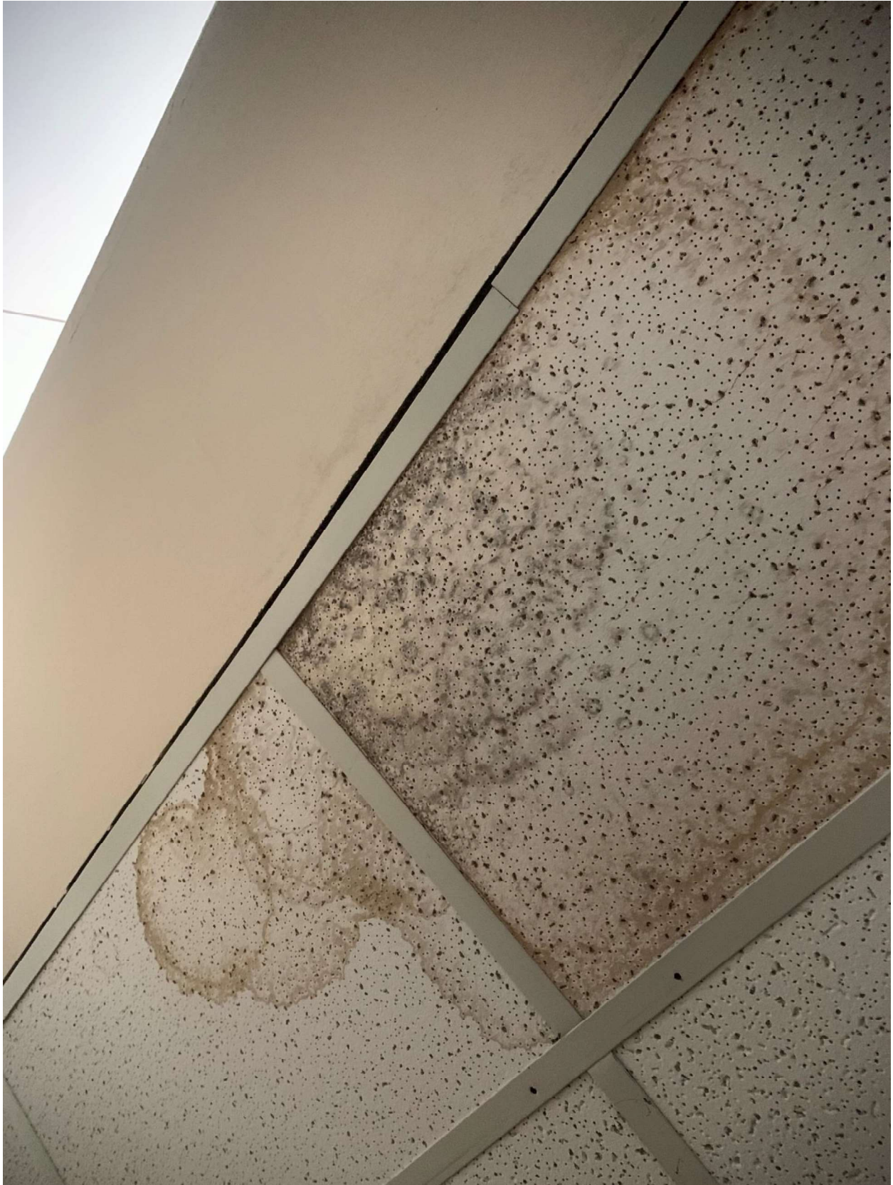
Figure 10 Suspended ceiling main floor
