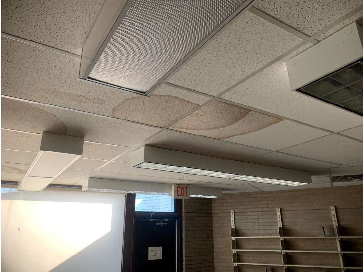
Figure 13 Suspended ceiling main floor
