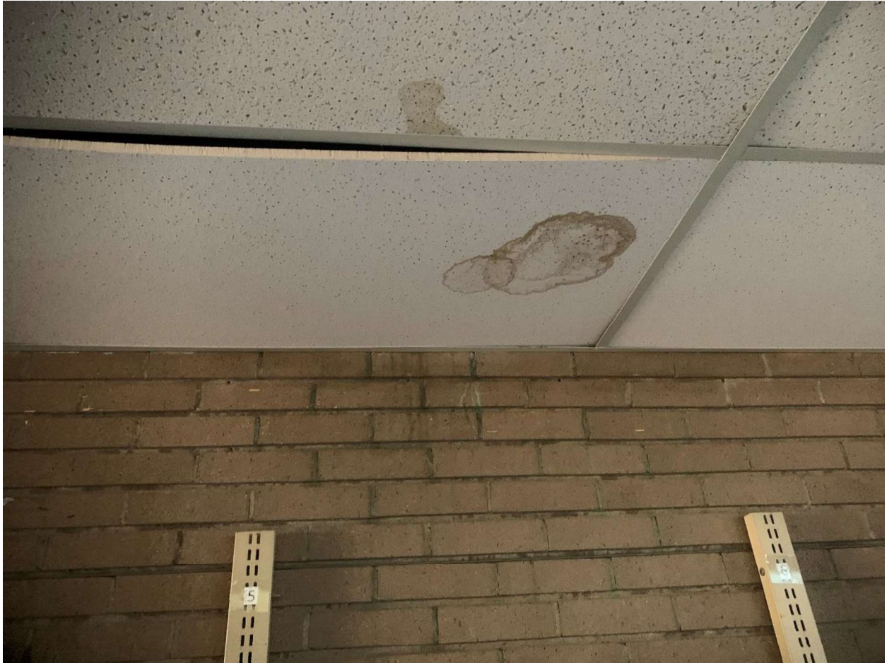
Figure 14 Suspended ceiling main floor
