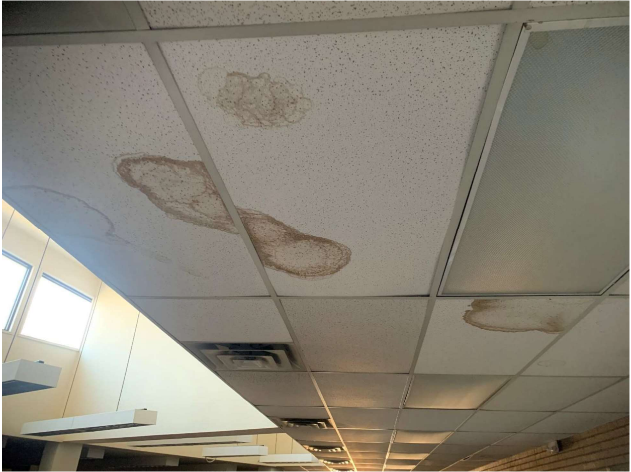
Figure 12 Suspended ceiling main floor
