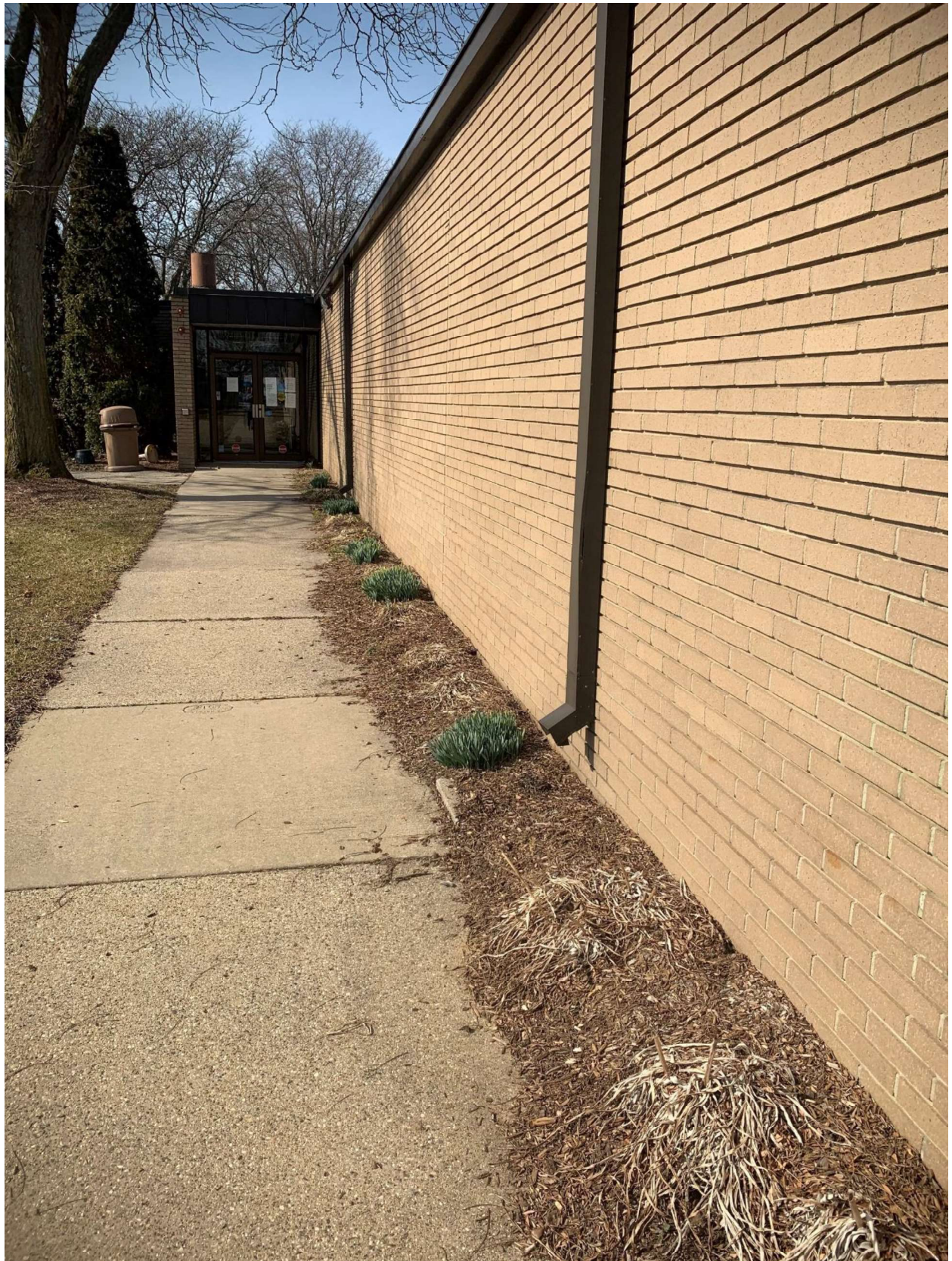
Figure 15 Downspouts south side
