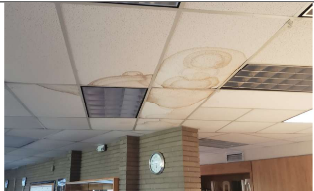
Lay-in ceiling, various areas of water damage
