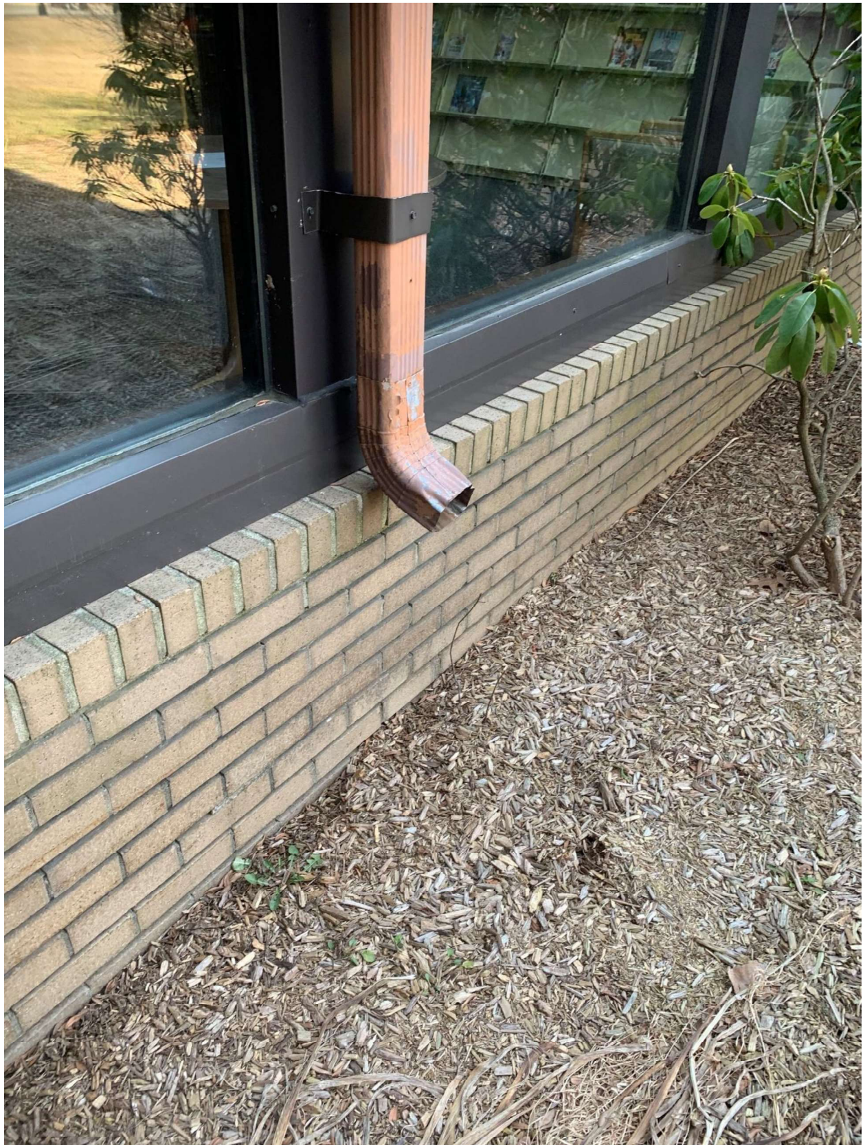
Figure 17 Downspout north side
