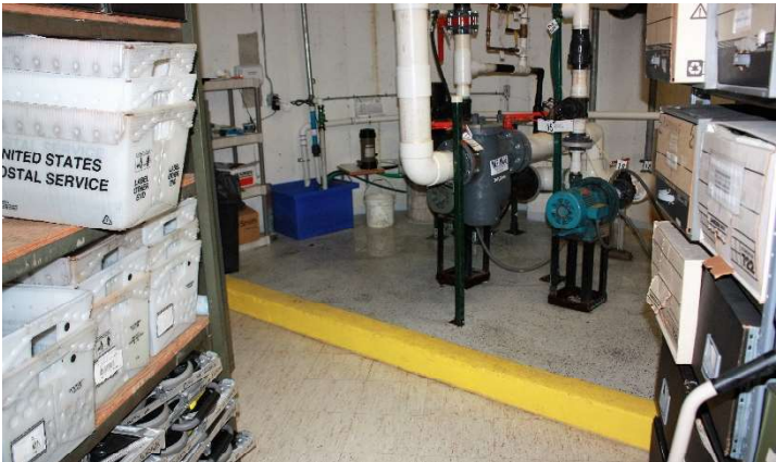
Basement Storage & Sump 2016
