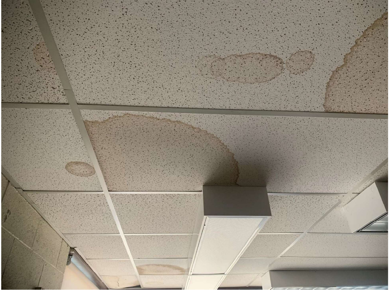
Figure 11 Suspended ceiling main floor
