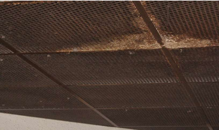
Fifth Floor Ventilation Grates 2013
