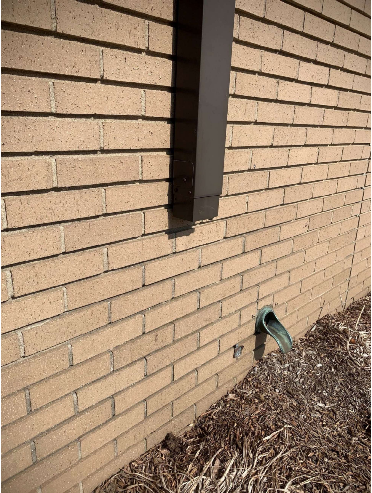
Figure 16 Downspout north side
