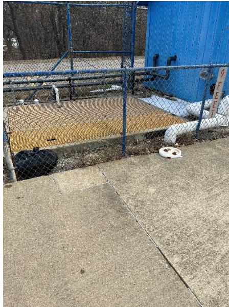
East Interior Fence
