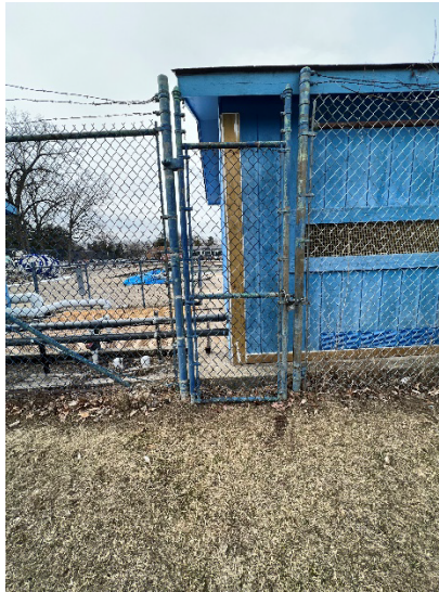
East Maintenance Gate
