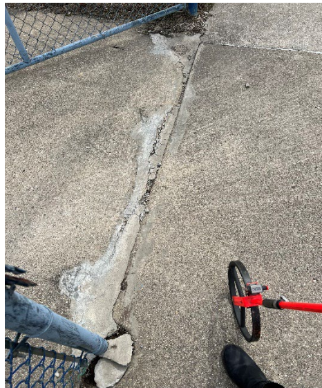
Concrete Replacement of East Entry Gate
