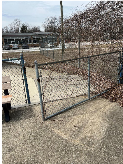
West Entry Gate
