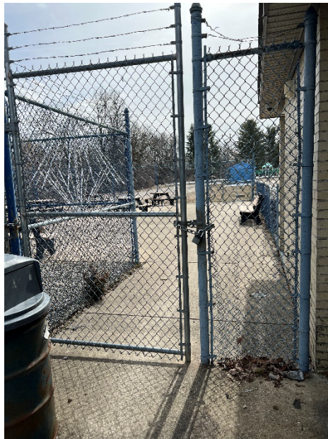
North Entry Gate- Will not be replaced with a gate, just fence.
