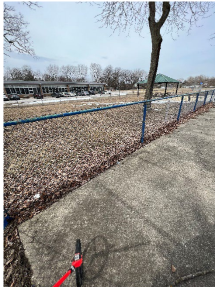
West Interior Fence Line
