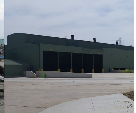
New Solid Waste Transfer & Processing Facility (After)
