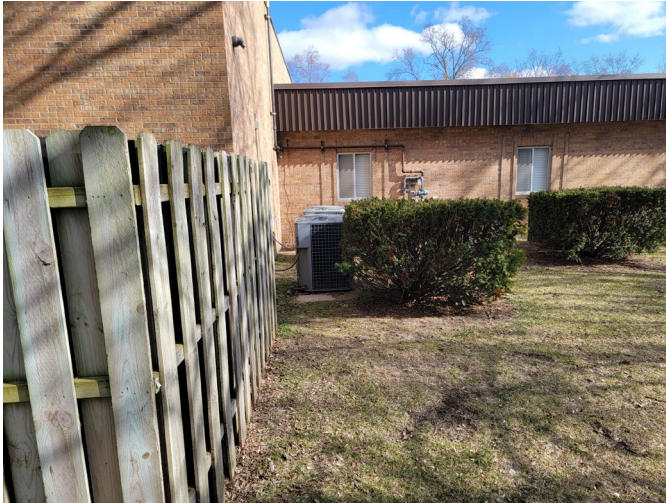
Figure 6: Existing NG Meter Location (side of Building) – Existing NG Generator Behind the Wood Fence/Screening
