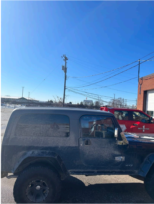
Figure 1: DTE Service Pole
