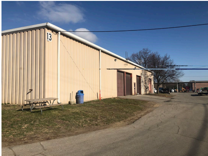
Figure 1: DPW Maintenance Building SE Corner
