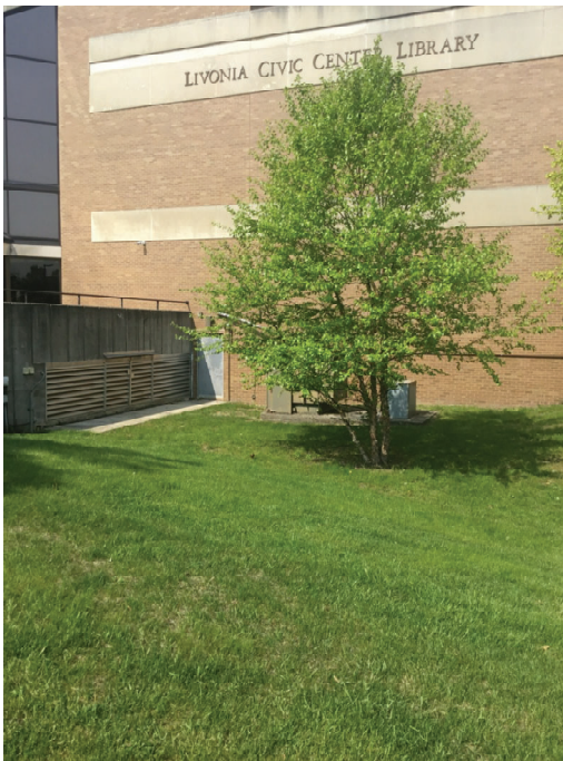
Areaway, access to lower level
