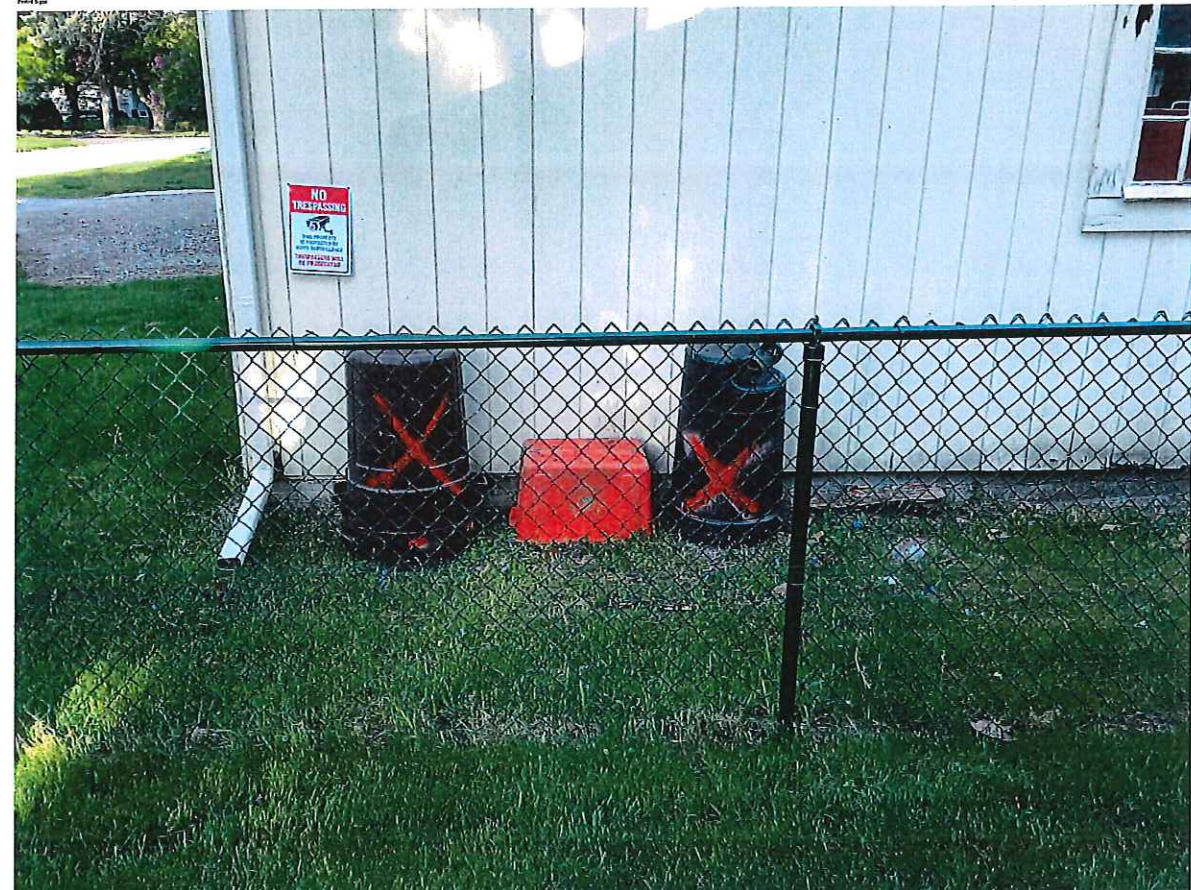
Concern on the corner of this property going to be not going any
