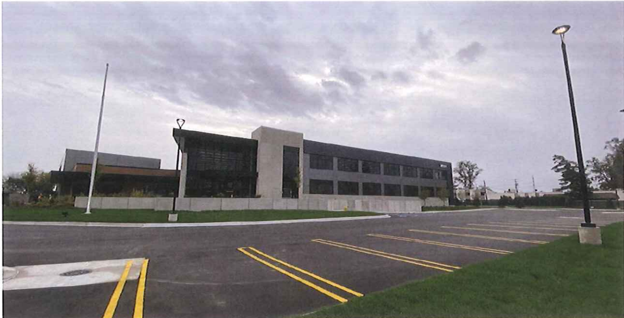
AFTER RENOVATION, OCTOBER 2023, FACING EAST TO FARMINGTON ROAD.
