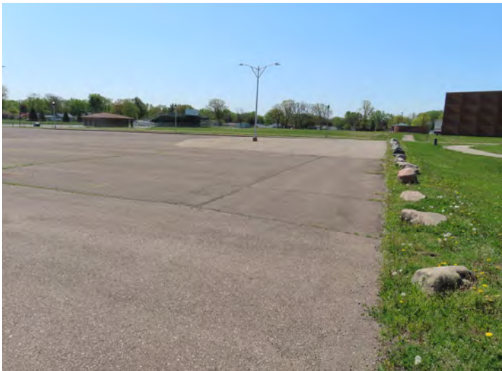
LOOKING SOUTHEAST AT PROPOSED LAND DIVISION FROM WEST 5 MILE ROAD
