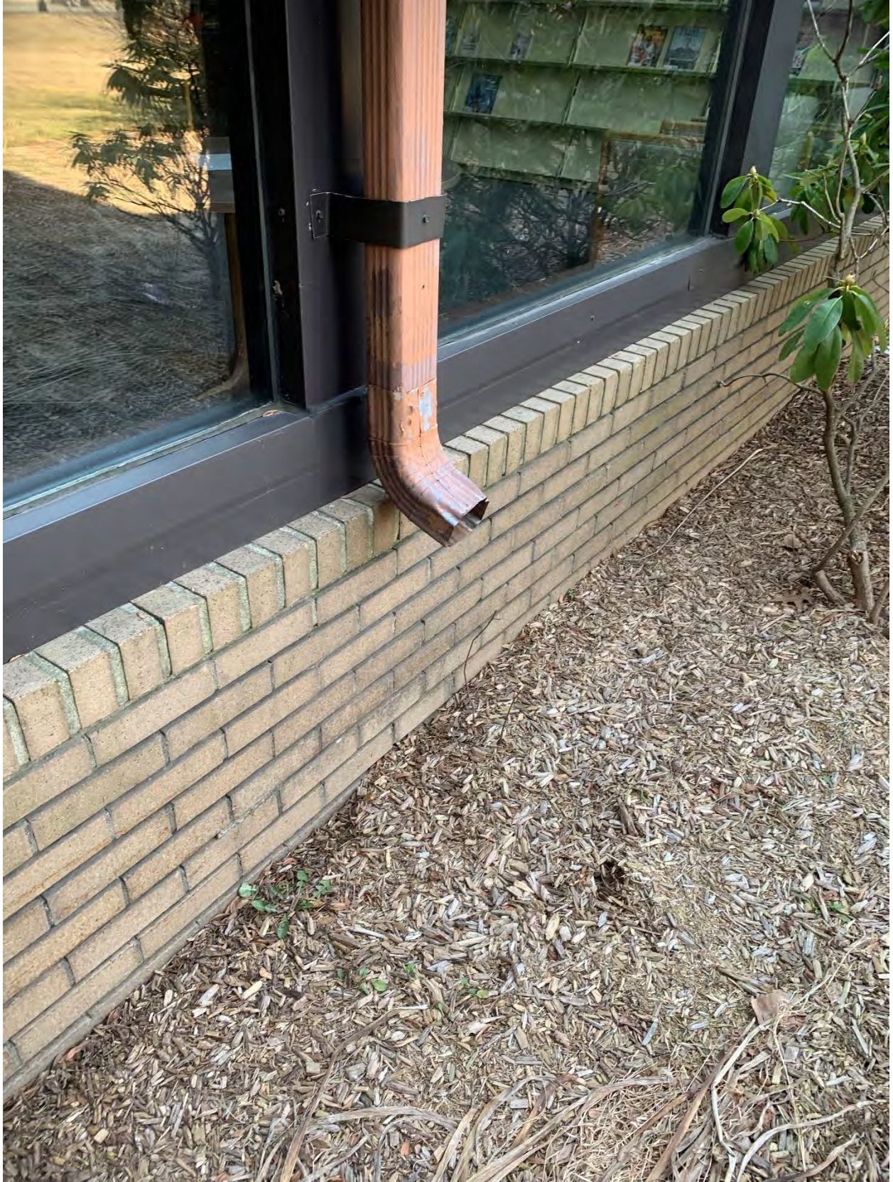
Figure 17 Downspout north side
