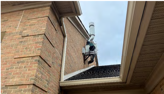
Façade and roof
