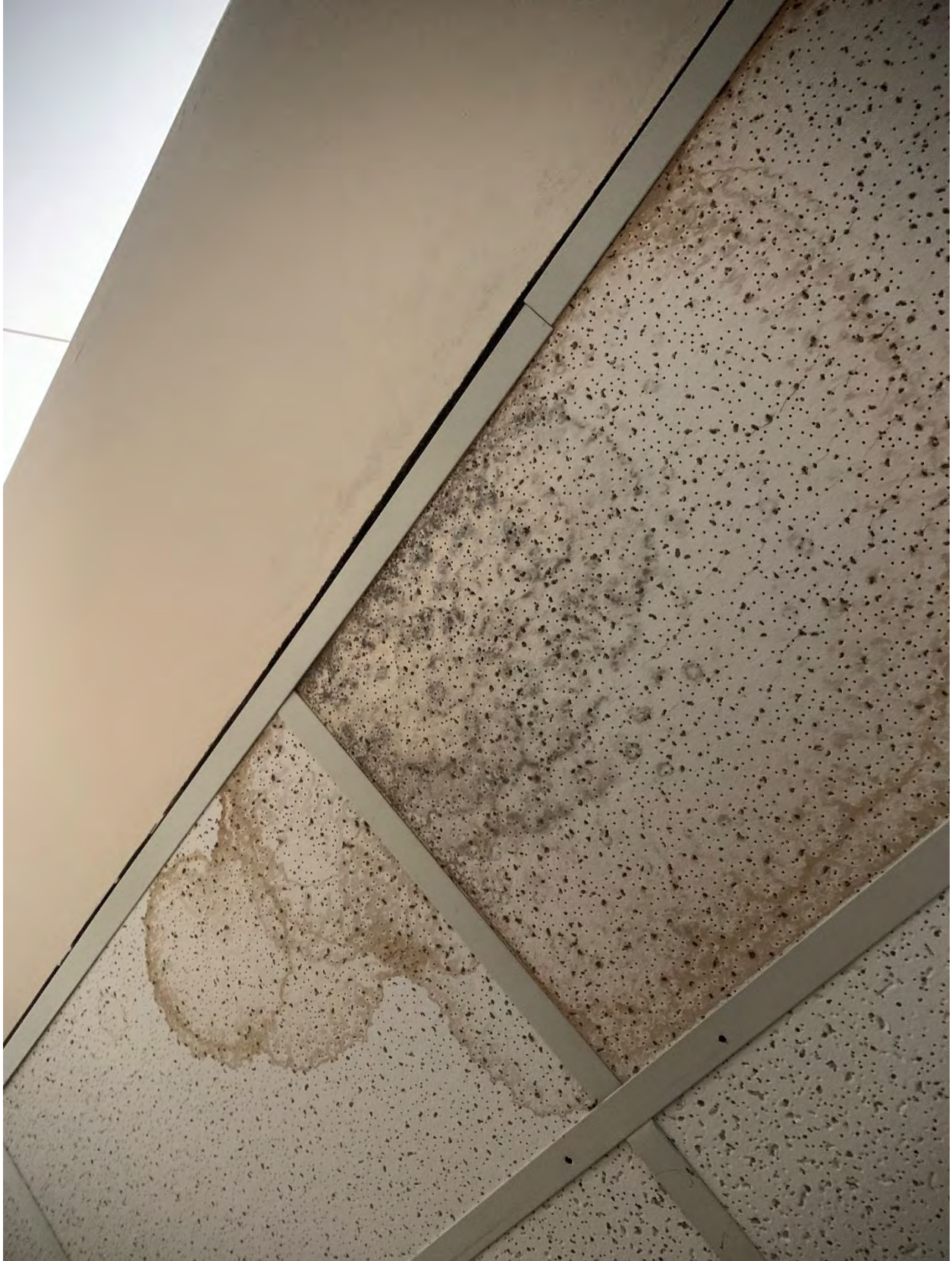
Figure 10 Suspended ceiling main floor
