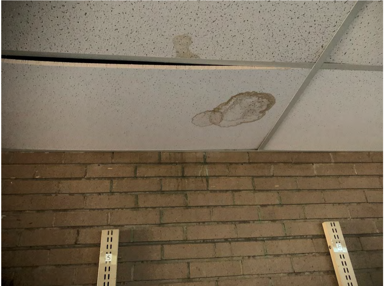
Figure 14 Suspended ceiling main floor
