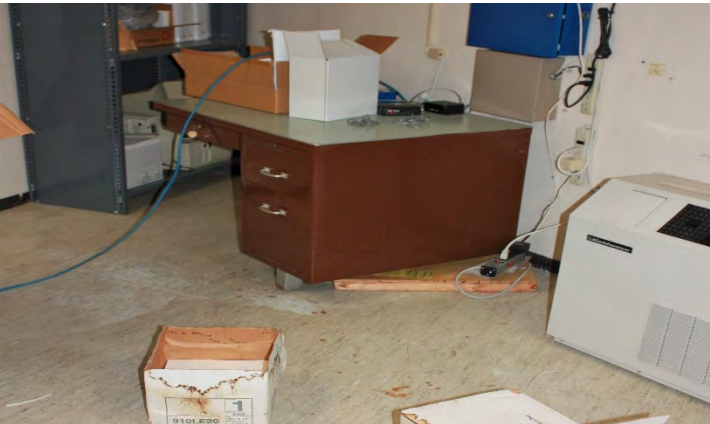
Phone Room Leak Aftermath
