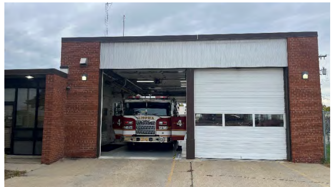
Apparatus bay doors
