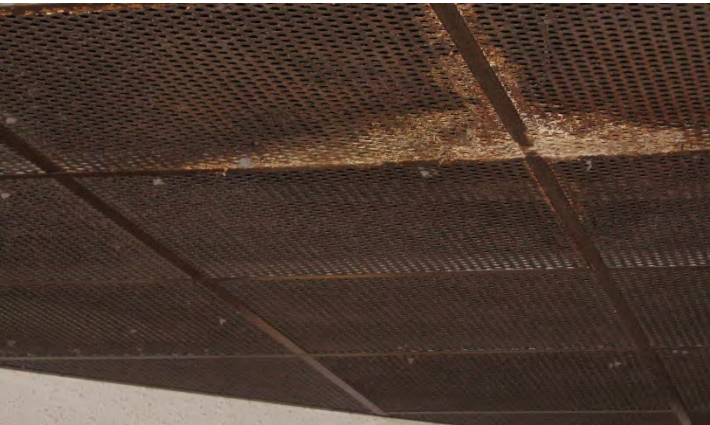
Fifth Floor Ventilation Grates 2013
