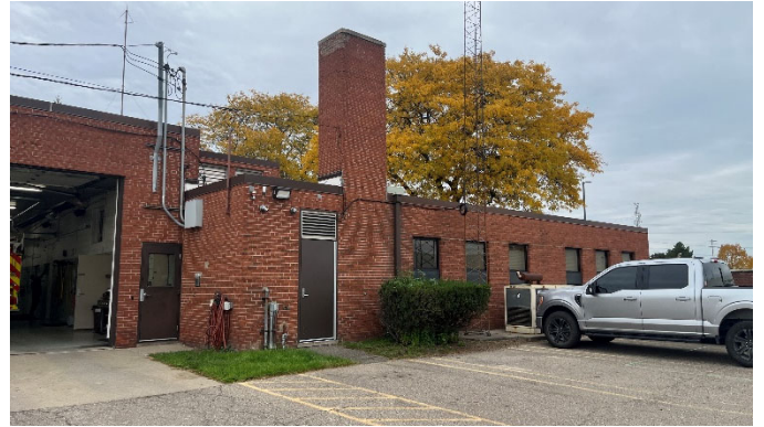
Asphalt parking lot
