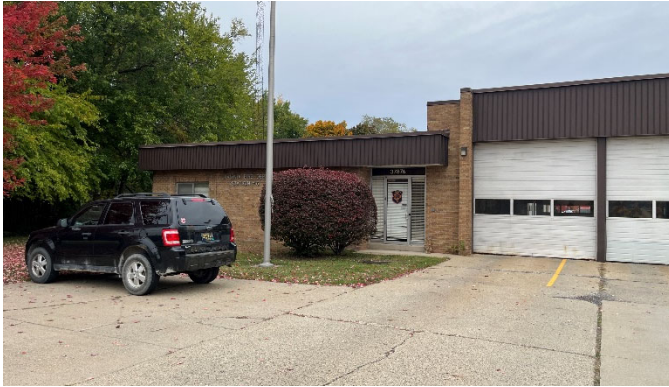
Entry and Apparatus Bay doors
