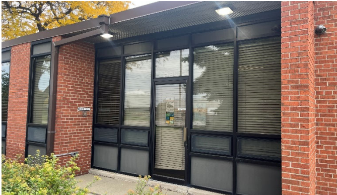
Uninsulated, single pane storefront
