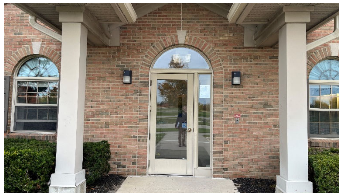
Facade and door
