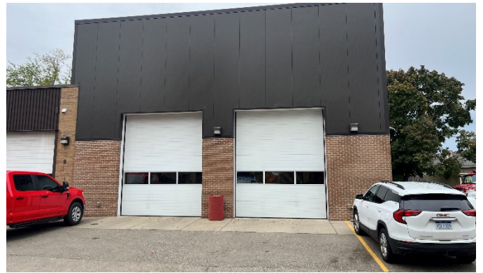
Apparatus Bay doors
