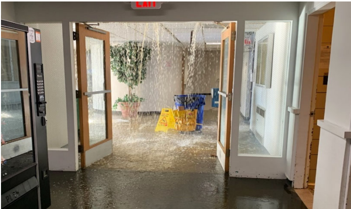
Ruptured Pipe in Annex 2022
