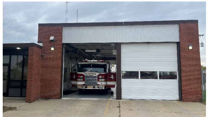
Apparatus bay doors
