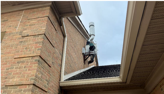
Façade and roof
