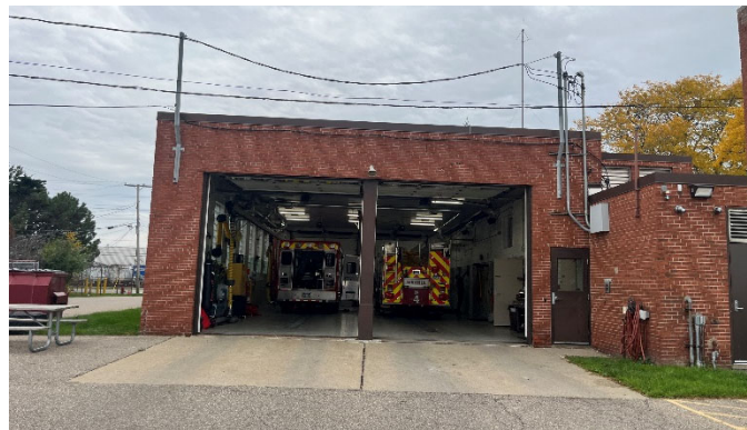
Facade and apparatus bay doors
