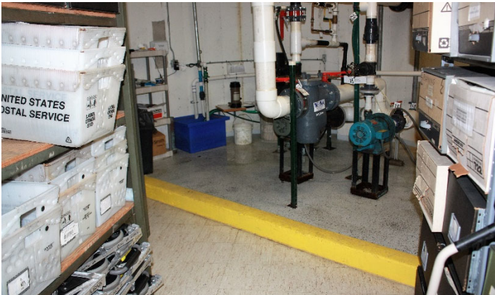
Basement Storage & Sump 2016
