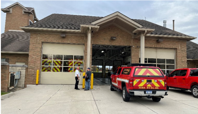
Parking lot and drive aisle
