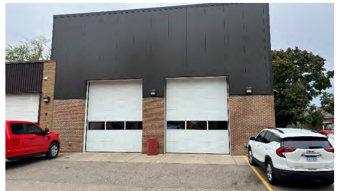
Apparatus Bay doors
