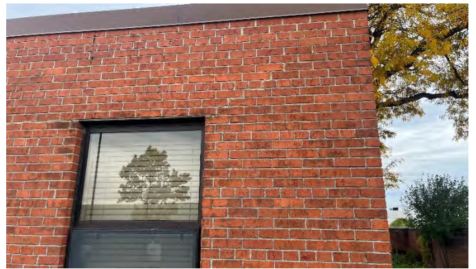
Facade and windows
