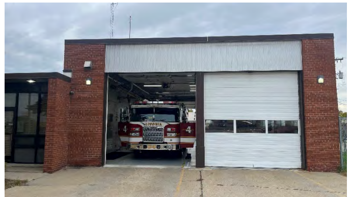
Apparatus bay doors
