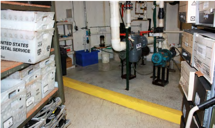
Basement Storage & Sump 2016
