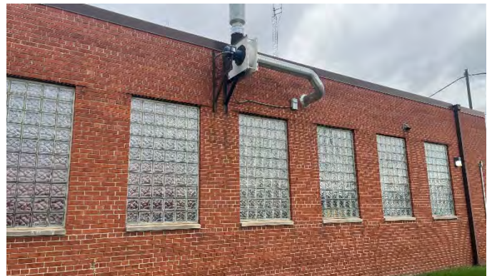
Glass block windows at Apparatus Bay
