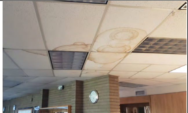
Lay-in ceiling, various areas of water damage
