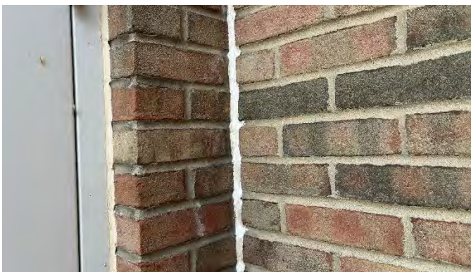
Caulking at control joint and door
