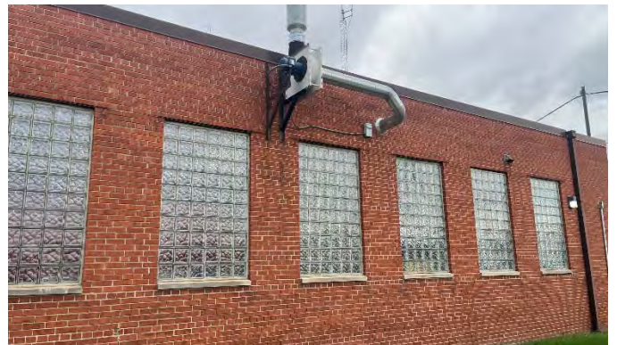
Glass block windows at Apparatus Bay
