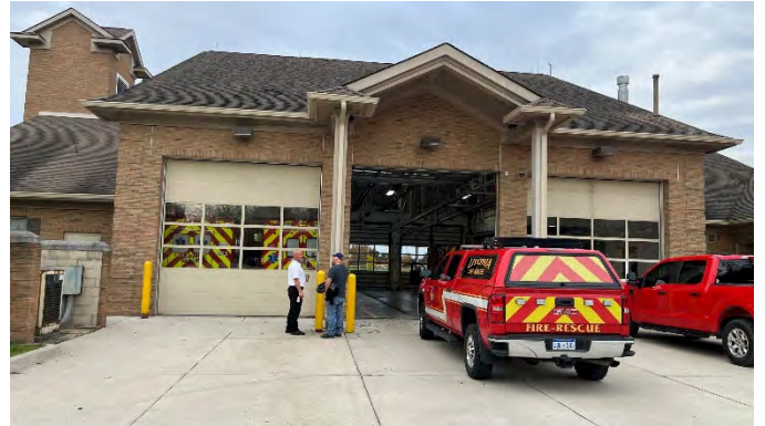
Façade and roof
