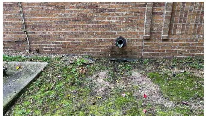
Overflow drain
