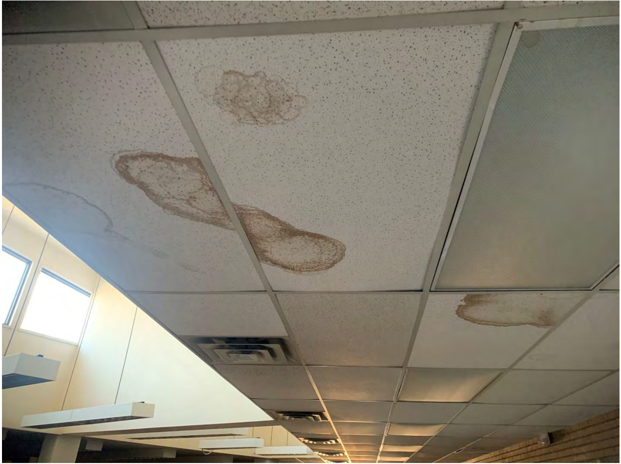
Figure 12 Suspended ceiling main floor
