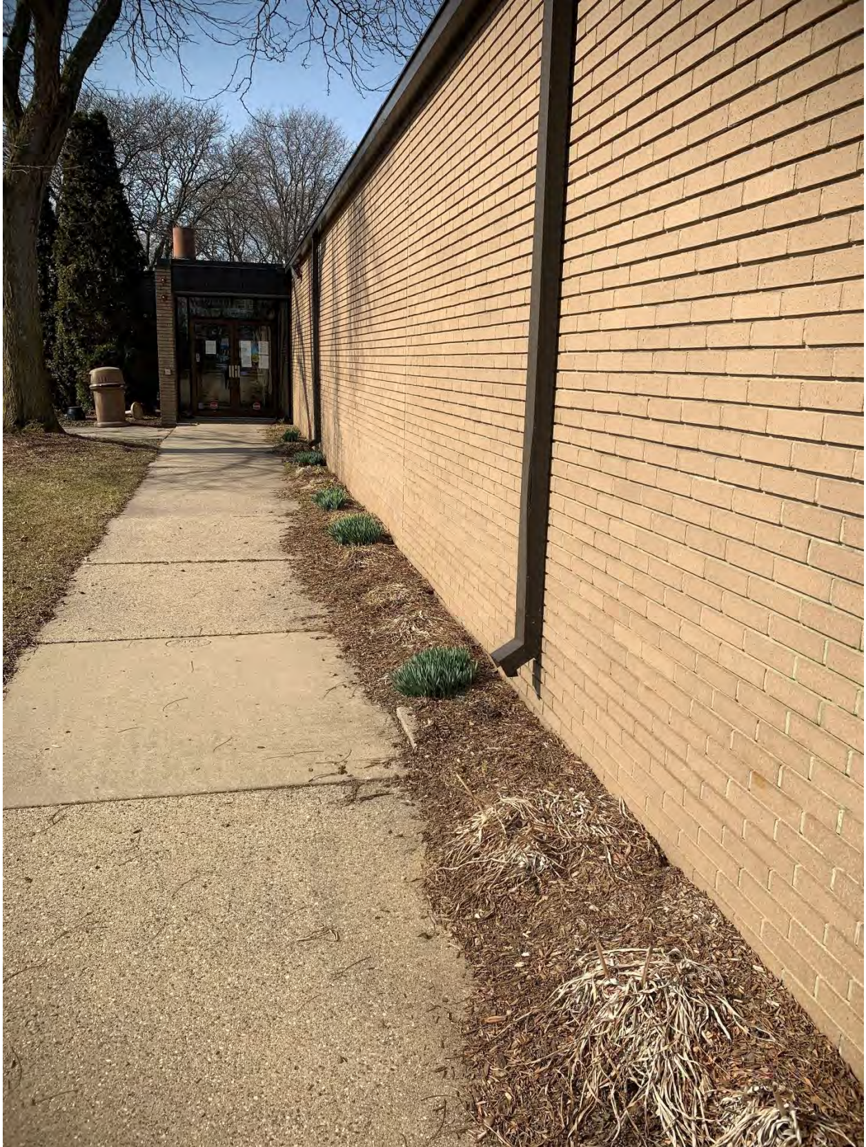
Figure 15 Downspouts south side
