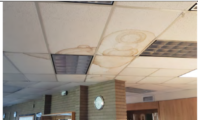
Lay-in ceiling, various areas of water damage
