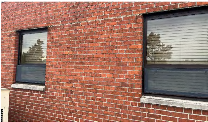
Facade and windows
