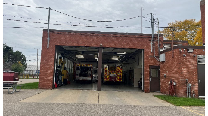
Facade and apparatus bay doors
