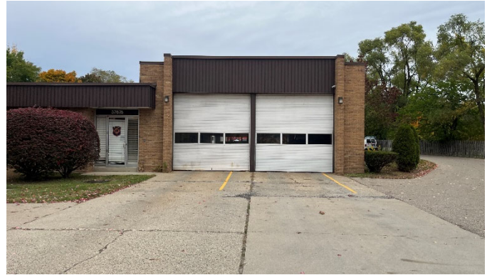
Entry and Apparatus Bay doors
