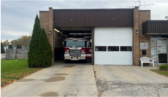
Apparatus bay doors
