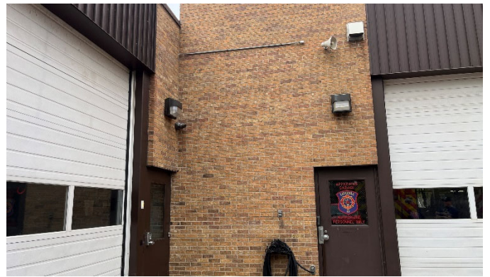
Apparatus bay doors
