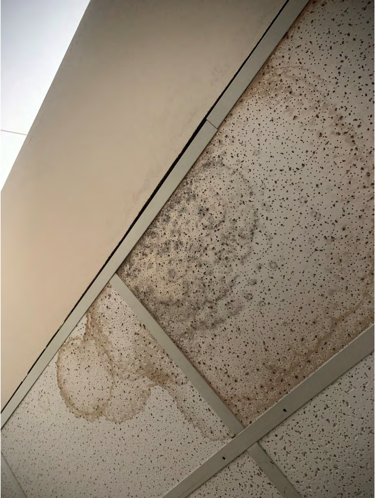
Figure 10 Suspended ceiling main floor
