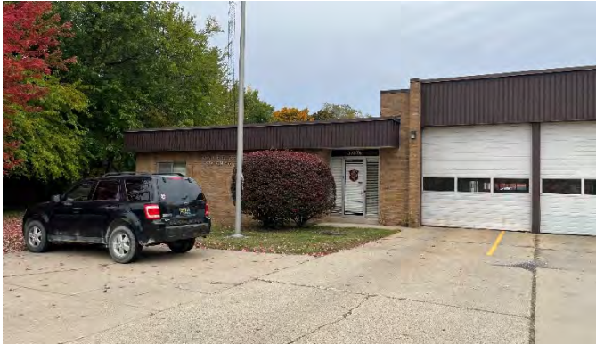
Entry and Apparatus Bay doors
