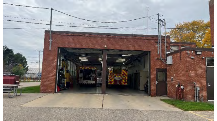
Facade and apparatus bay doors
