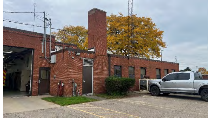
Asphalt parking lot
