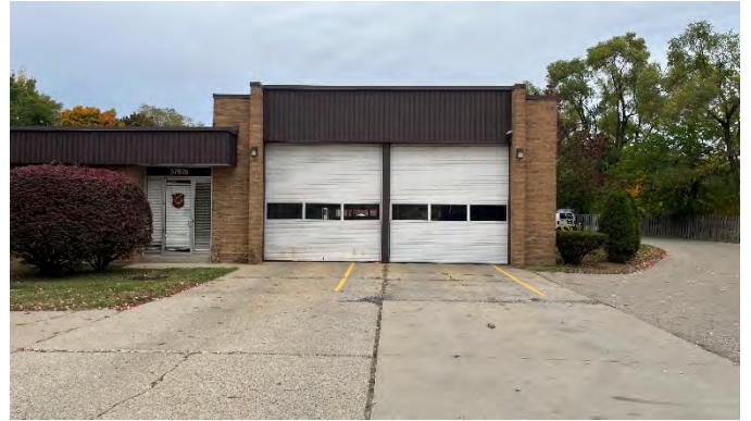
Entry and Apparatus Bay doors
