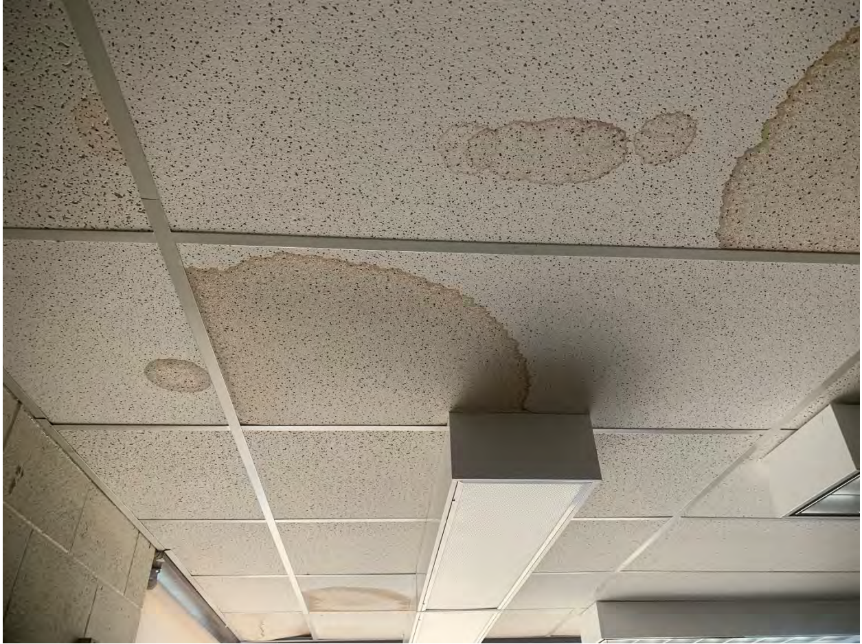
Figure 11 Suspended ceiling main floor
