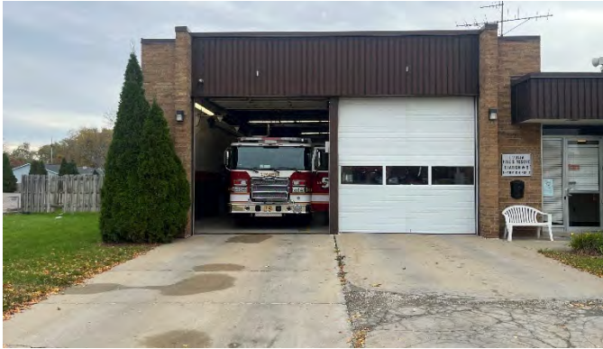
Apparatus bay doors
