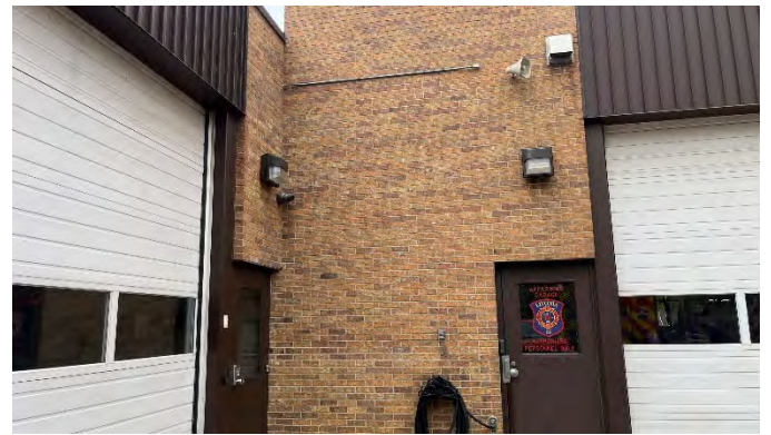
Apparatus bay doors
