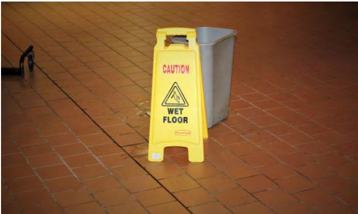
First Floor Leak
