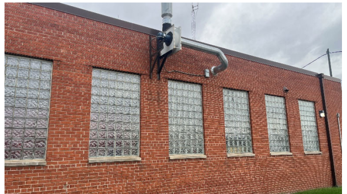
Glass block windows at Apparatus Bay
