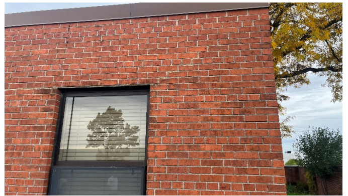
Facade and windows
