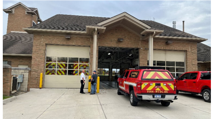
Façade and roof
