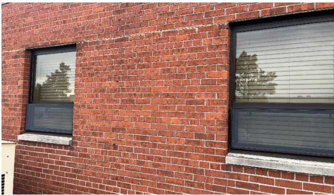
Facade and windows
