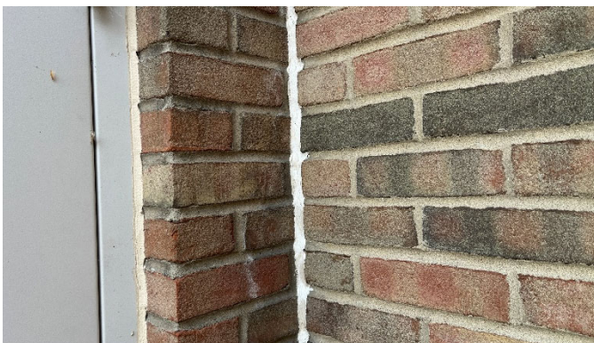
Caulking at control joint and door
