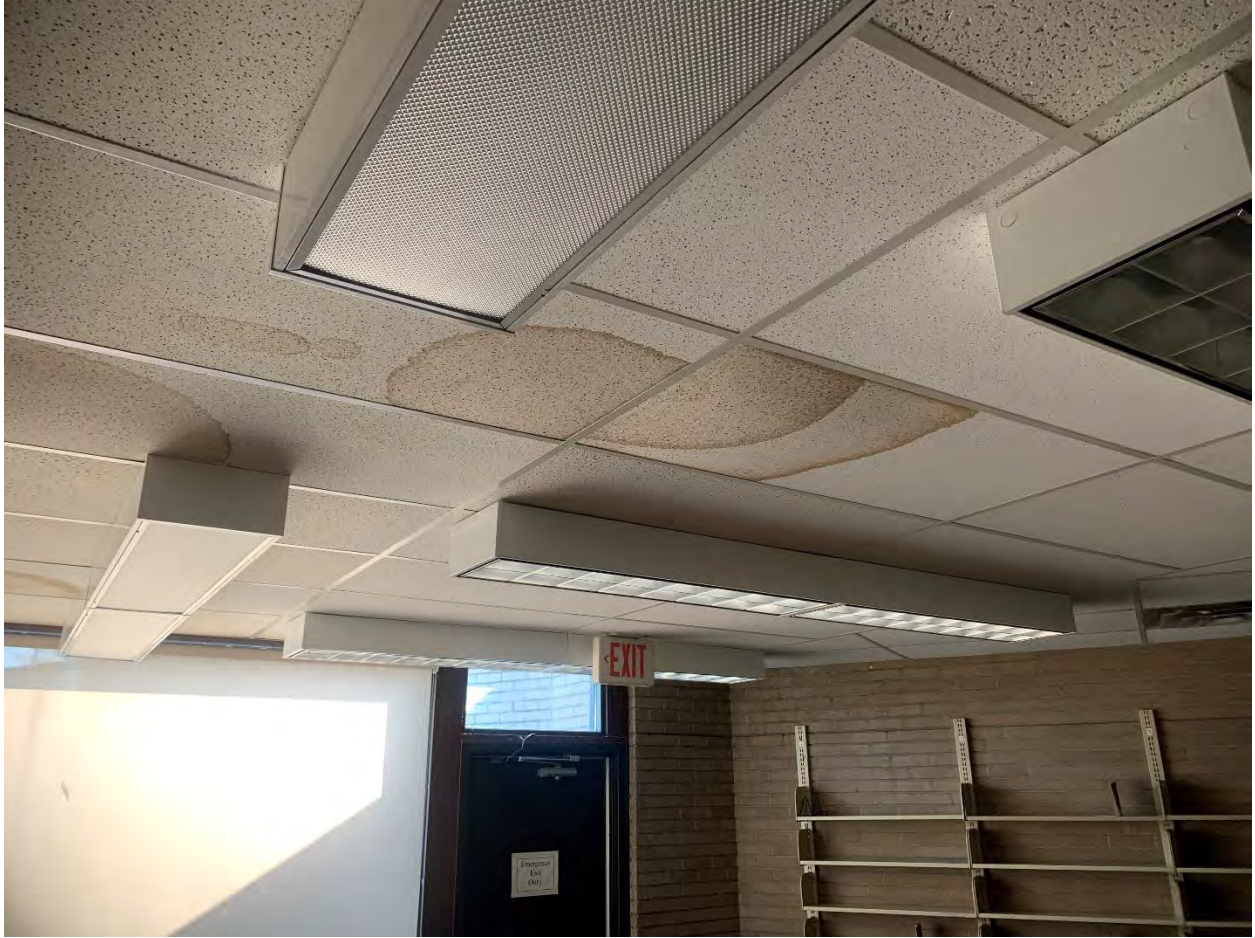
Figure 13 Suspended ceiling main floor
