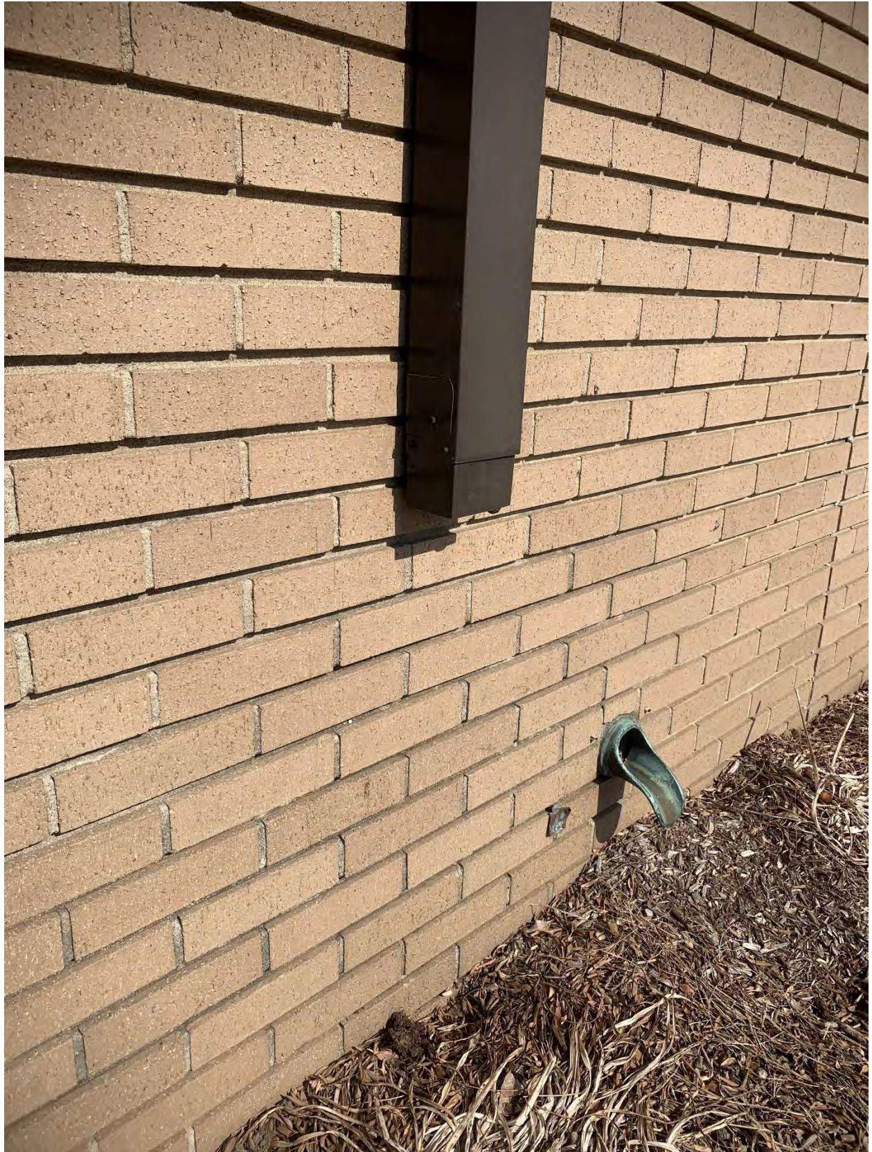
Figure 16 Downspout north side
