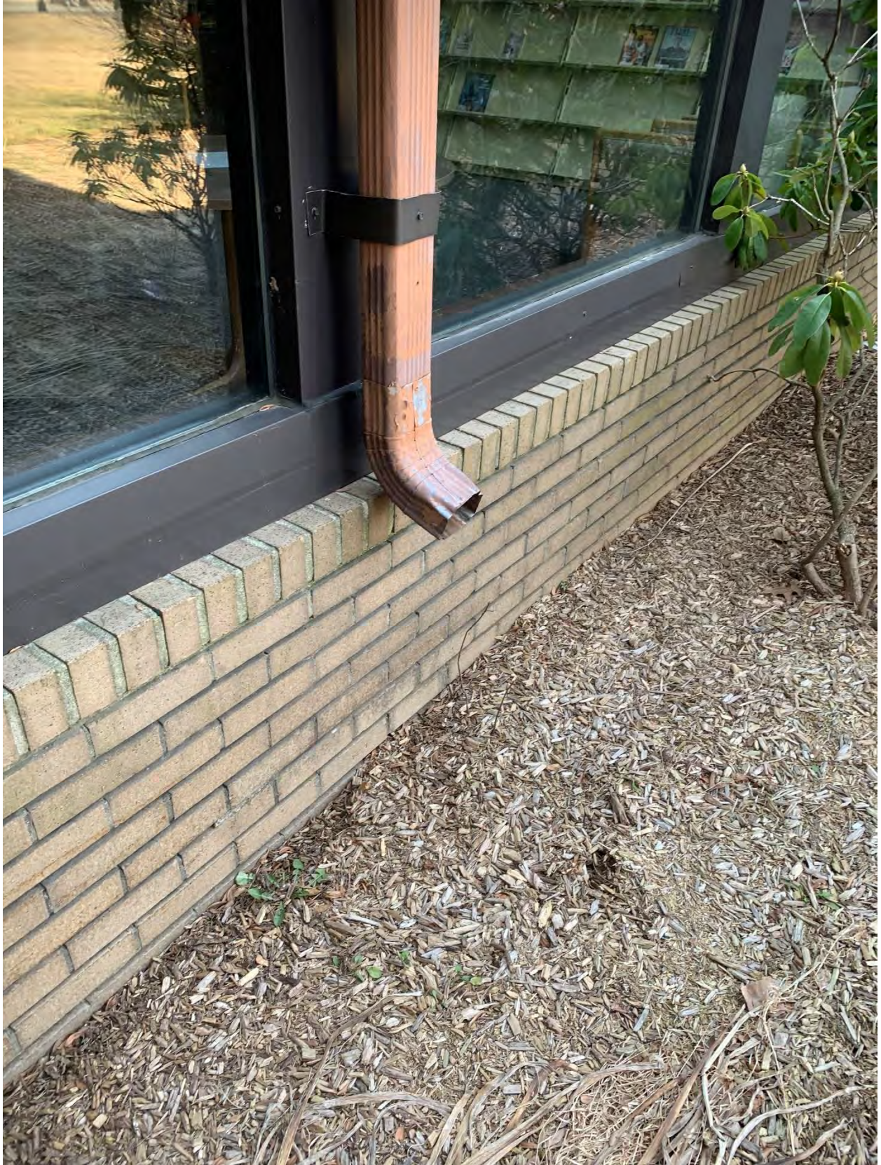
Figure 17 Downspout north side
