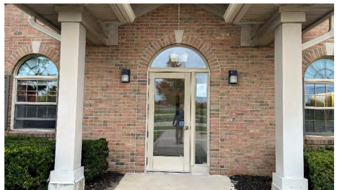
Facade and door
