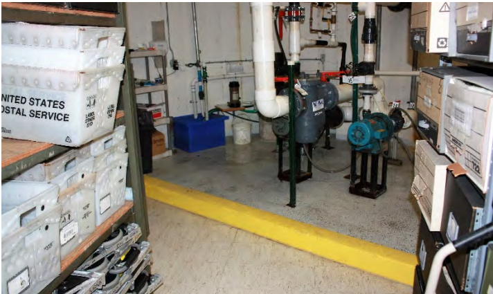
Basement Storage & Sump 2016
