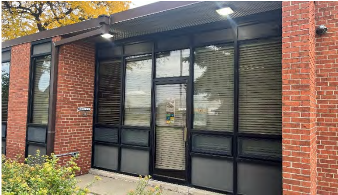
Uninsulated, single pane storefront
