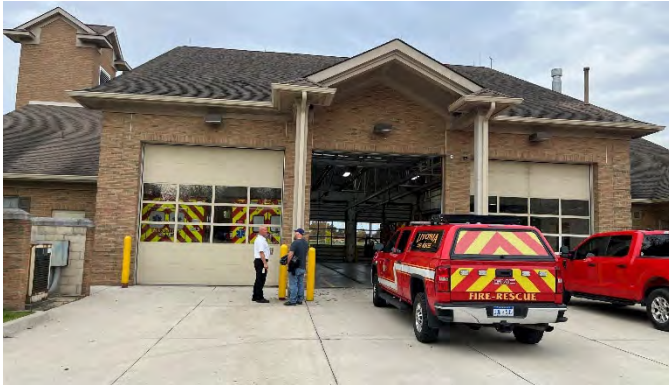
Parking lot and drive aisle
