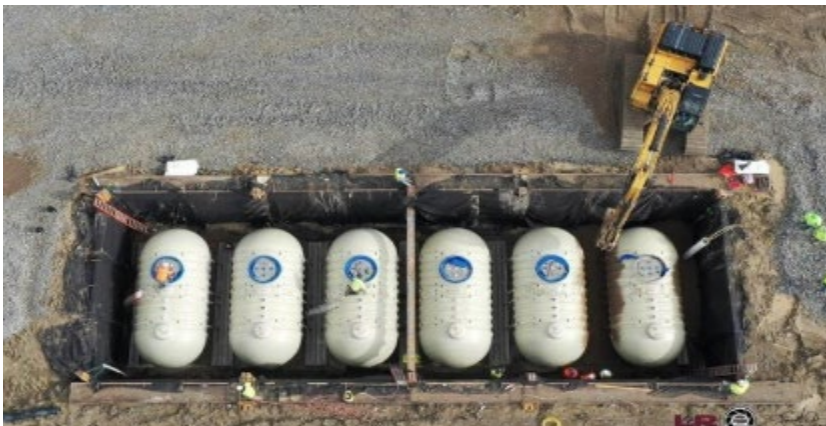
Picture above is from a Sheetz 6 storage tank installation
