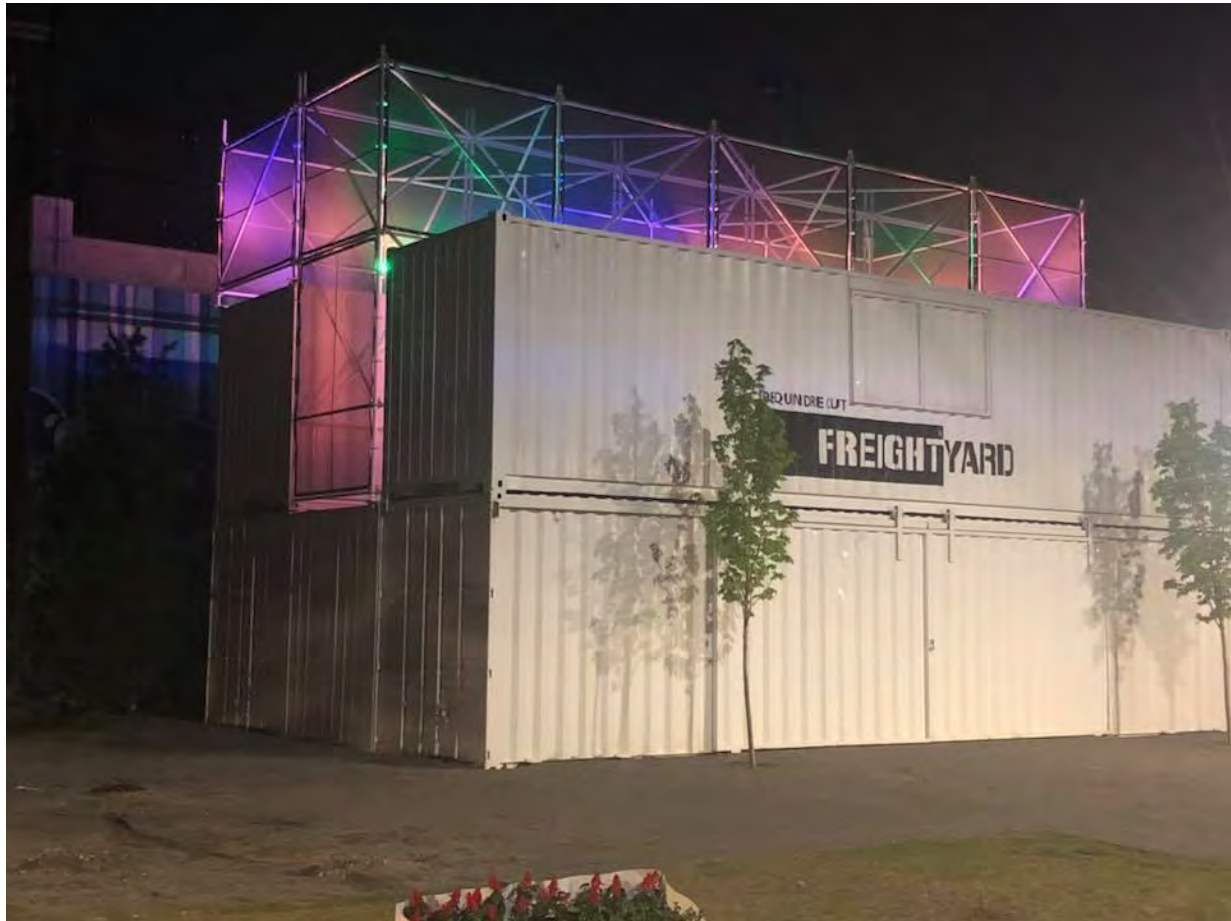
ABOVE: The “Hub” of the Freight Yard seen at night after hours. The Hub is comprised of five, 40 foot containers as well as a network of standard construction scaffolding, which facilitates accent lighting and event lighting and sound equipment.
