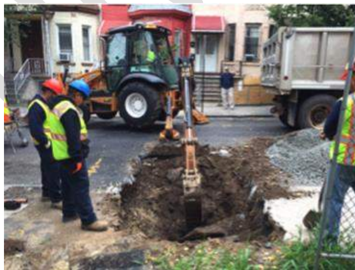
Figure 6: Method of Replacement - Open Cut
