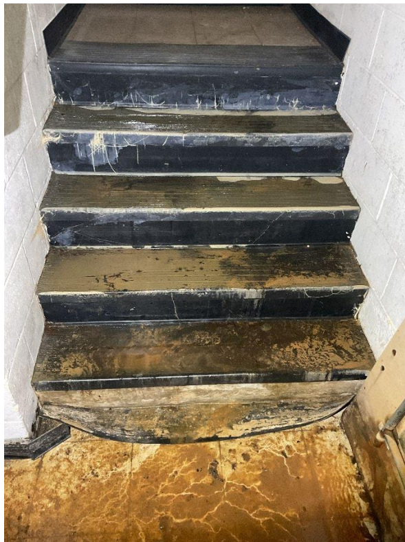
Basement – Kicker plate (Photo No. 4691)
