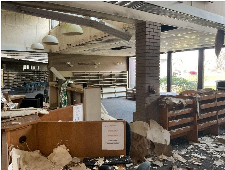
Main Floor – Floor conditions (2) (Photo No. 4975)
