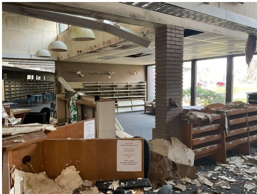
Main Floor – Floor conditions (2) (Photo No. 4975)
