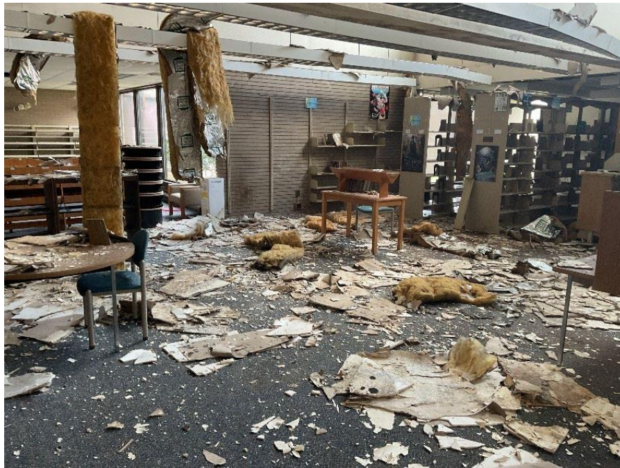
Main Floor – Floor conditions (Photo No. 4967)
