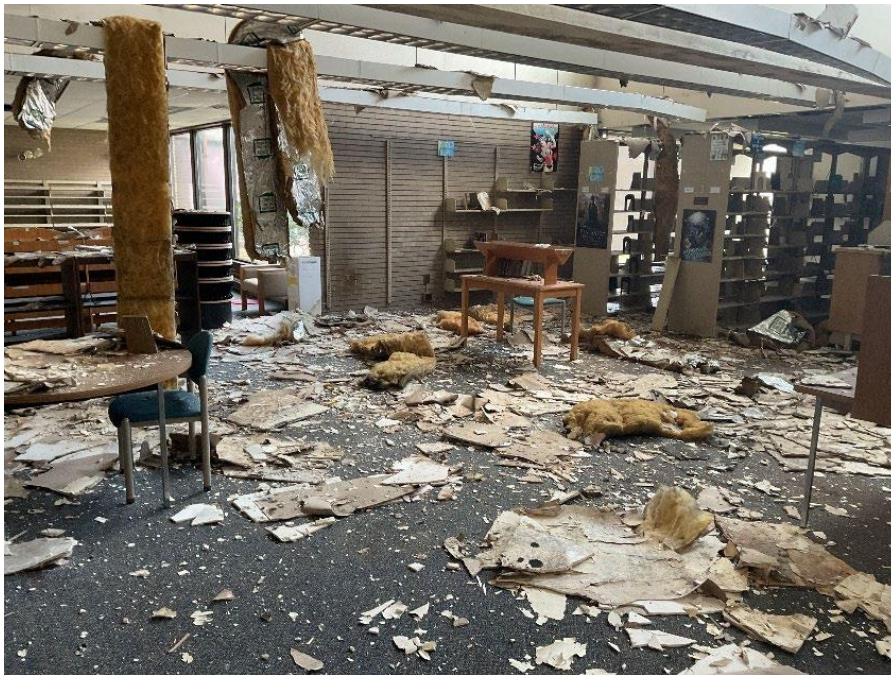
Main Floor – Floor conditions (Photo No. 4967)
