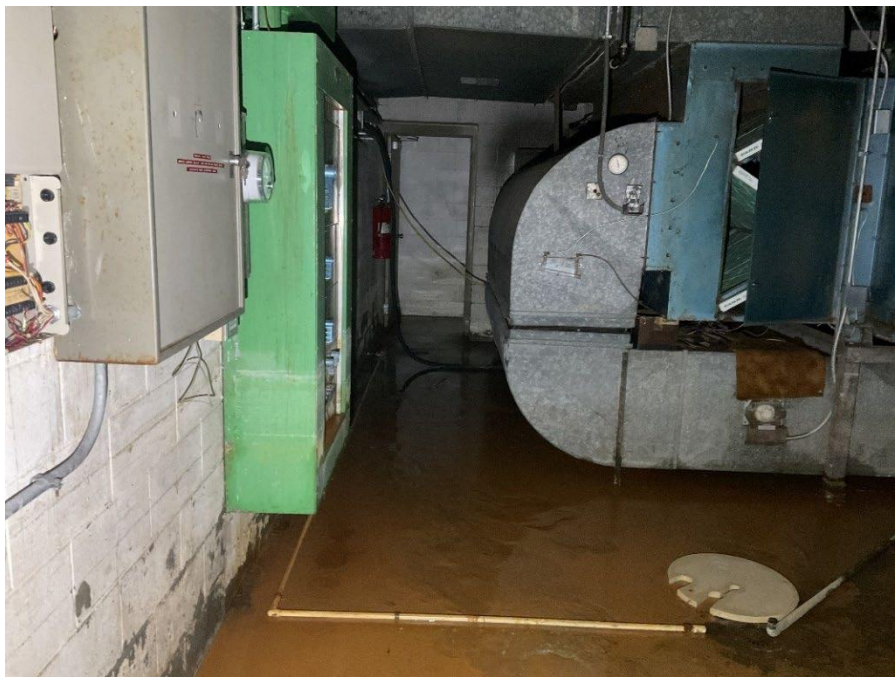
Basement – Mechanical Room floor (Photo No. 4723)
