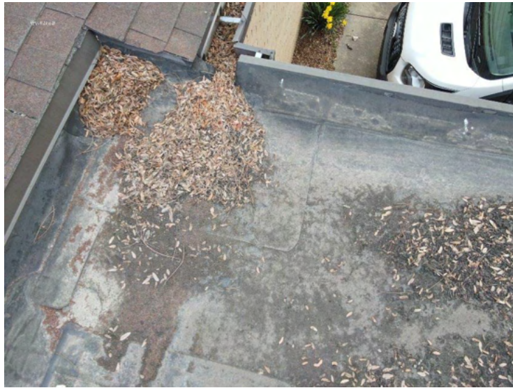
Flat Roof – Stockpile with tree leaves (Parking Lot Side Photo No. 1)
