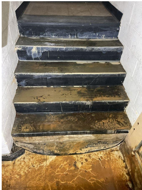
Basement – Kicker plate (Photo No. 4691)
