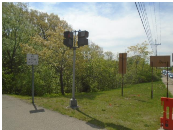
Parcel Looking Southeast
