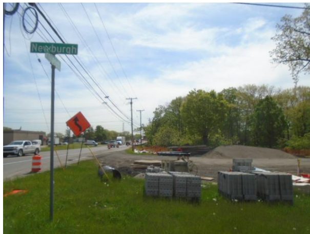
Parcel Looking East
