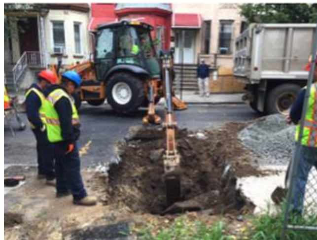
Figure 6: Method of Replacement - Open Cut
