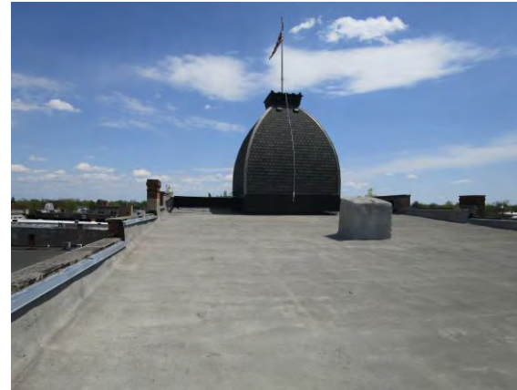
Figure 32 - View of the roof looking east at the Cupola.
