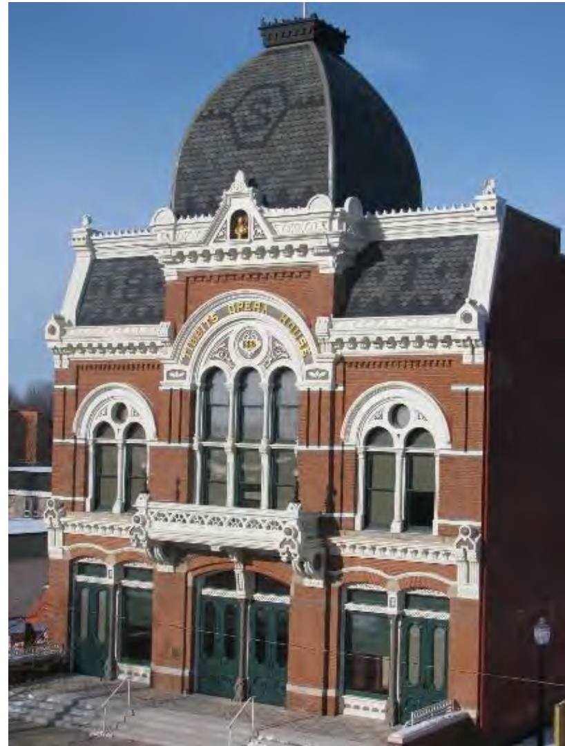
Figure 33 - View of the east elevation; the main façade and primary entrance to the Tibbits Opera House.
