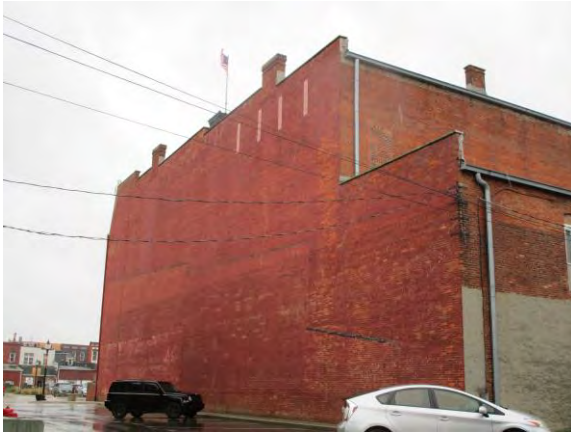
Figure 36 -View of the north elevation.
