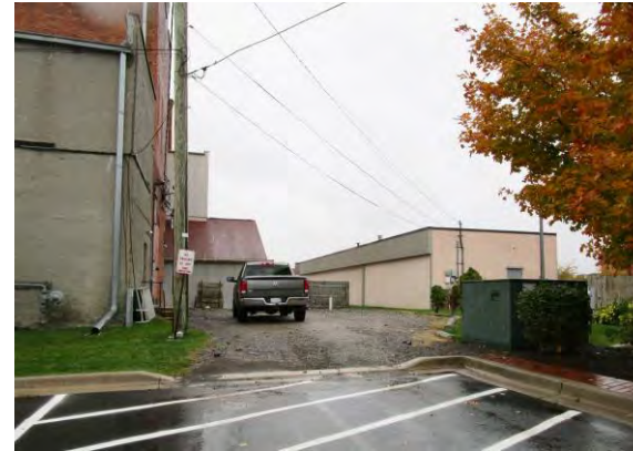
Figure 31 - View of the southwest corner of the building and existing loading dock and transformer.
