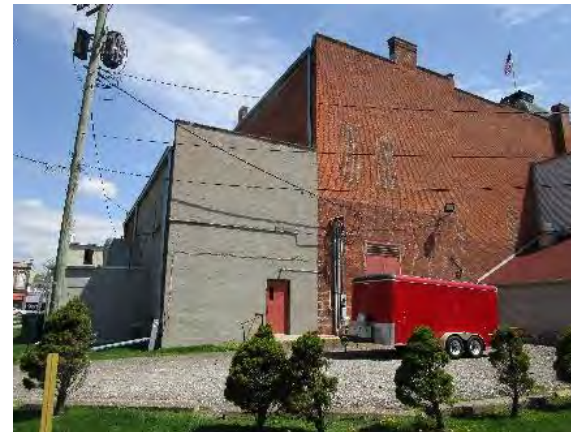
Figure 38 - View of the southwest façade.
