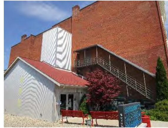
Figure 37 - View of the southeast façade.
