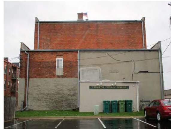
Figure 35 - View of the west elevation.
