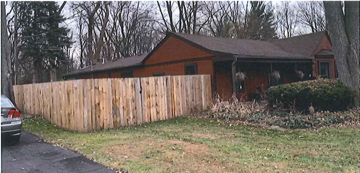
Figure 3 - View of property from W
