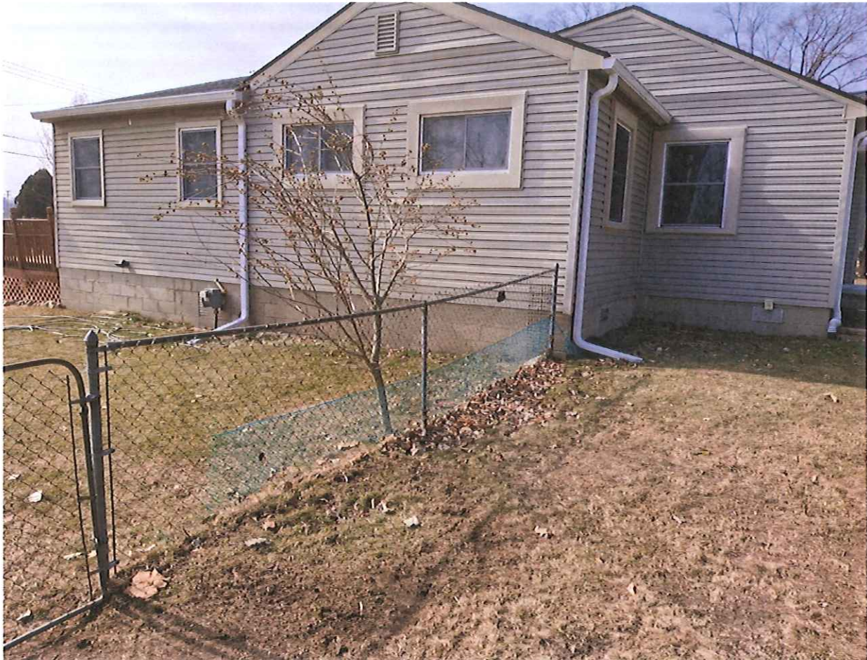
Existing Chain Link Fence:
